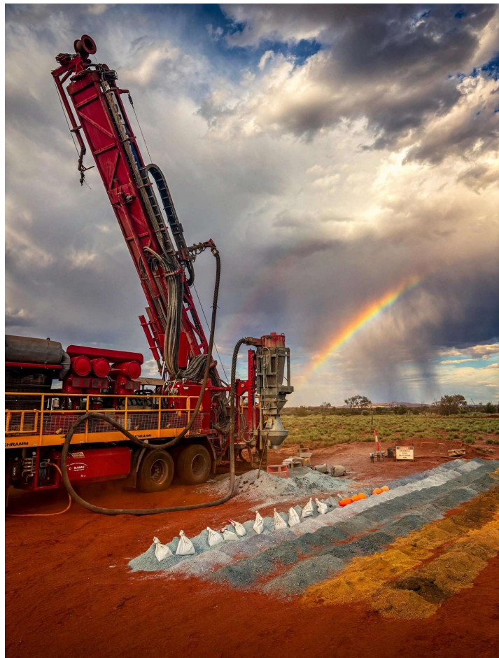
Figure 1: Drill Rig on Site at Southwest
