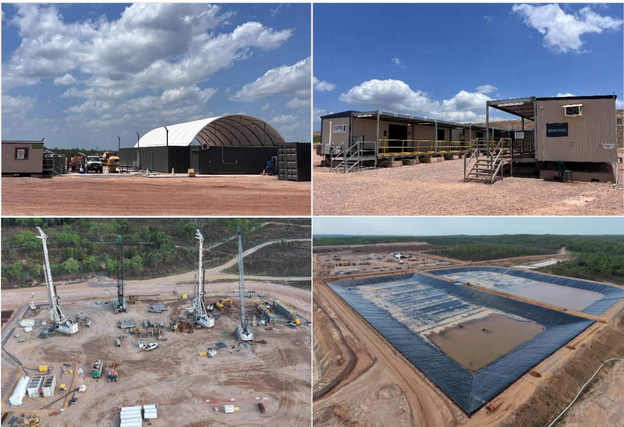
Figure 5 Infrastructure works at BP33 (clockwise from top left) 1. Contractor laydown area with mobile maintenance facility 2. Site offices 3. Completed mine water dam cells 4. Ventilation shafts development works
