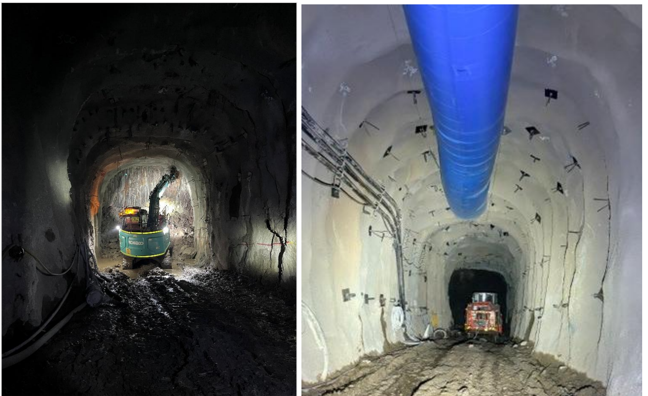
Figure 8 BP33 underground decline development
