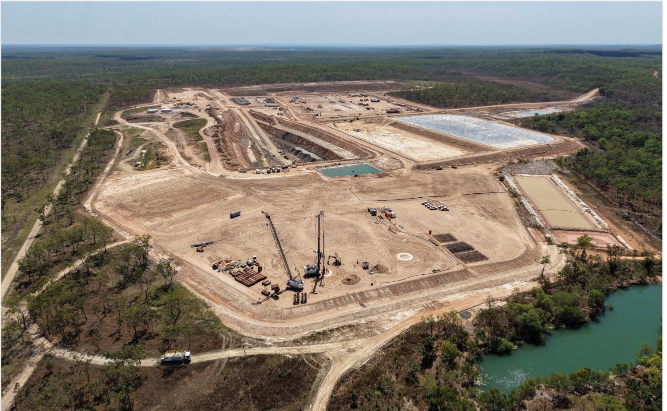
Figure 7 BP33 site overview with ventilation shaft development including piling works in the foreground
