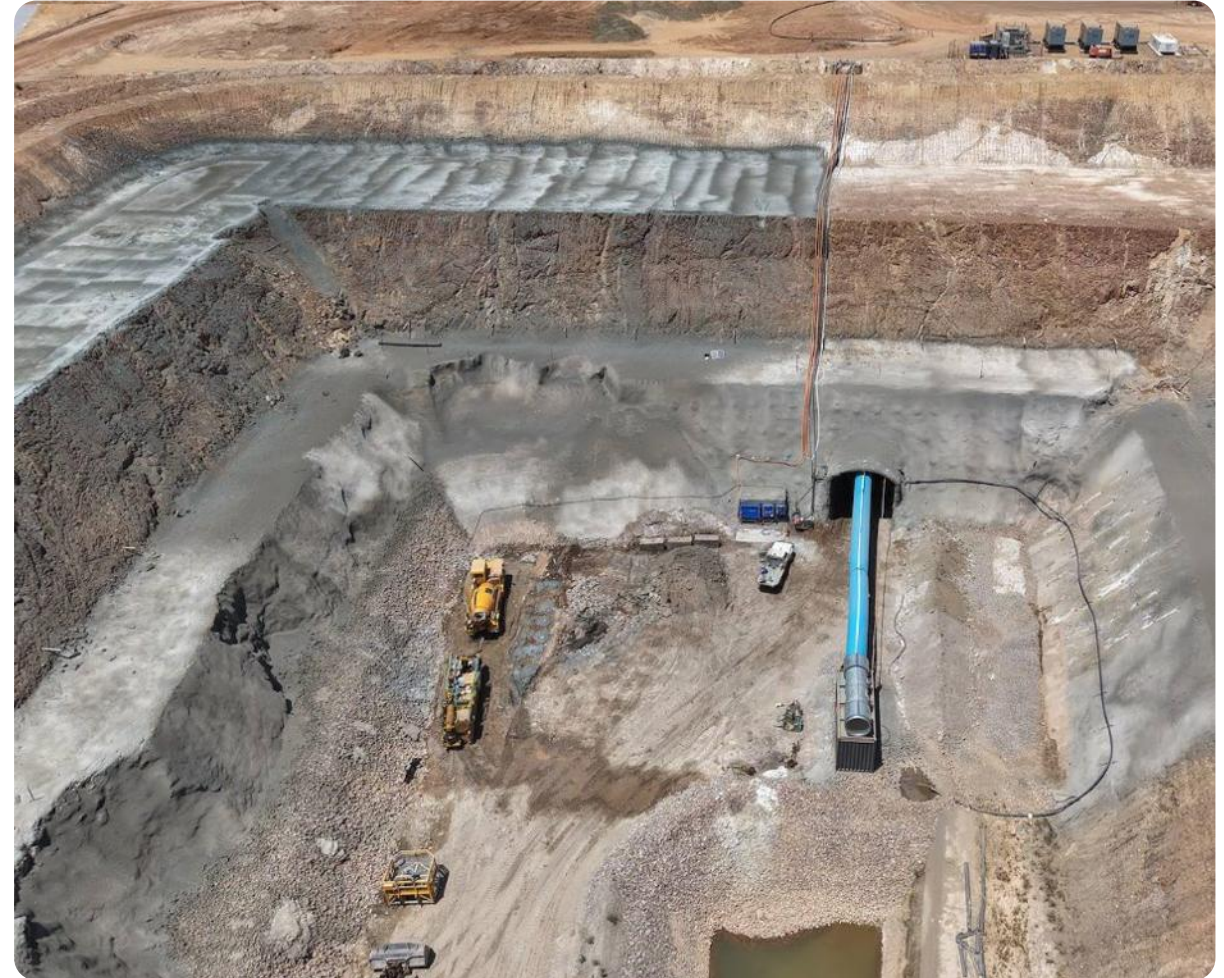
BP33 underground development progress, including box cut remediation, completed portal and temporary ventilation fan
