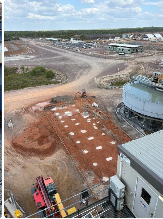
DMS plant brownfields modifications (Left to right) 1. Upgraded rolls crusher screen. 2. Reflux classifier pad. 3. New middlings conveyor
