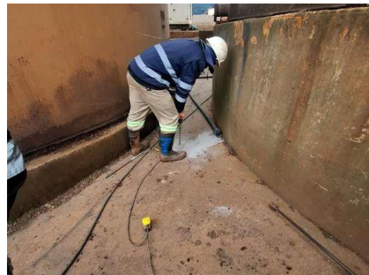
Drilling of Pre-Oxidation surface beds to allow for DCP testing of underlaying layer works.
