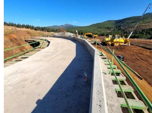
Visual post-concrete inspection of the stacker wall bund wall.
