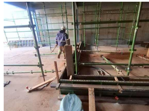
Pre-concrete inspection of Gold room bund wall area.
