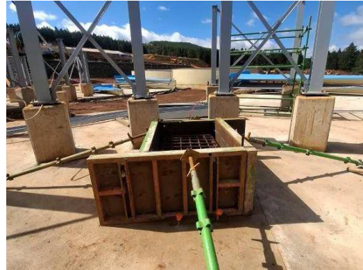
Pre-concrete shutter inspection of pump bases at Thickener 1000.
