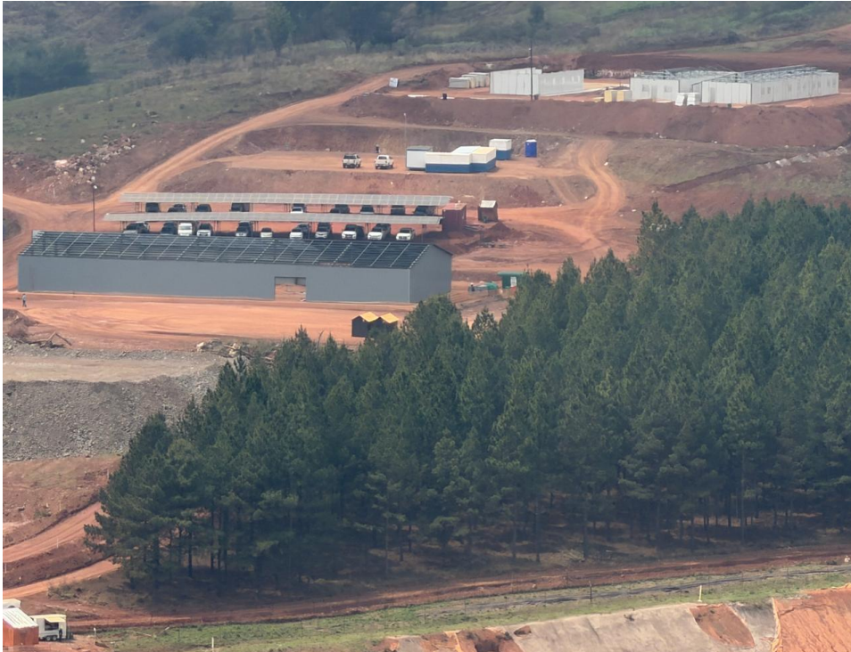
Management Offices, Solar Carpark, Goods shed
