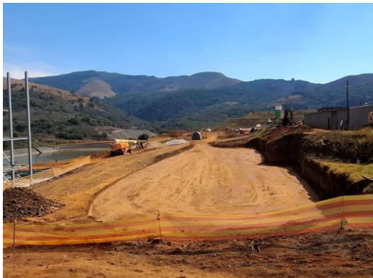
Area 800 Stabilenka installation completed and backfilled.
