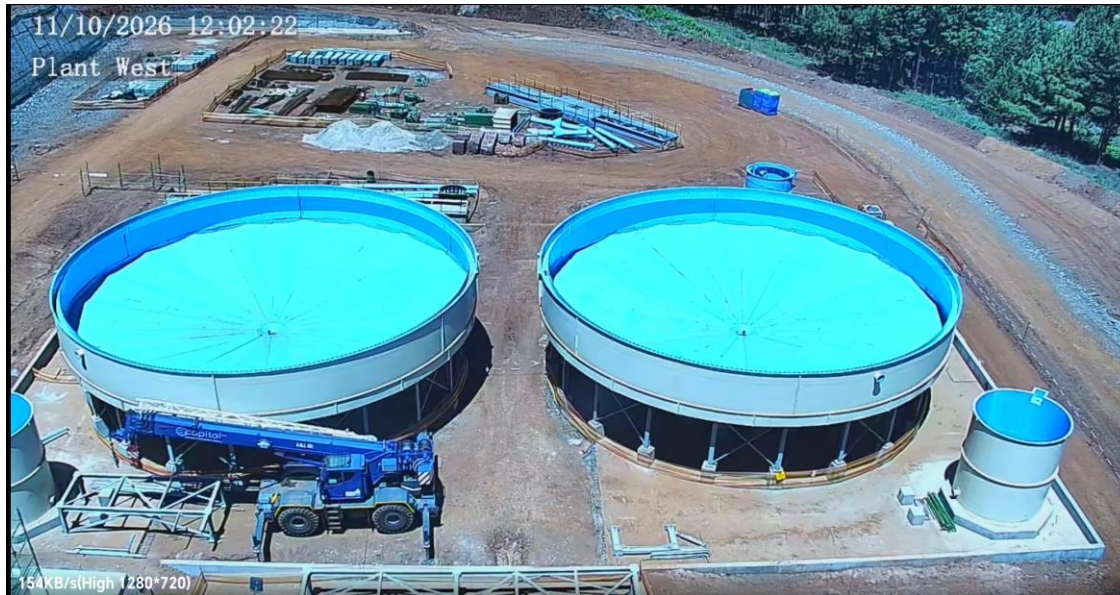
Thicker Tanks being constructed
