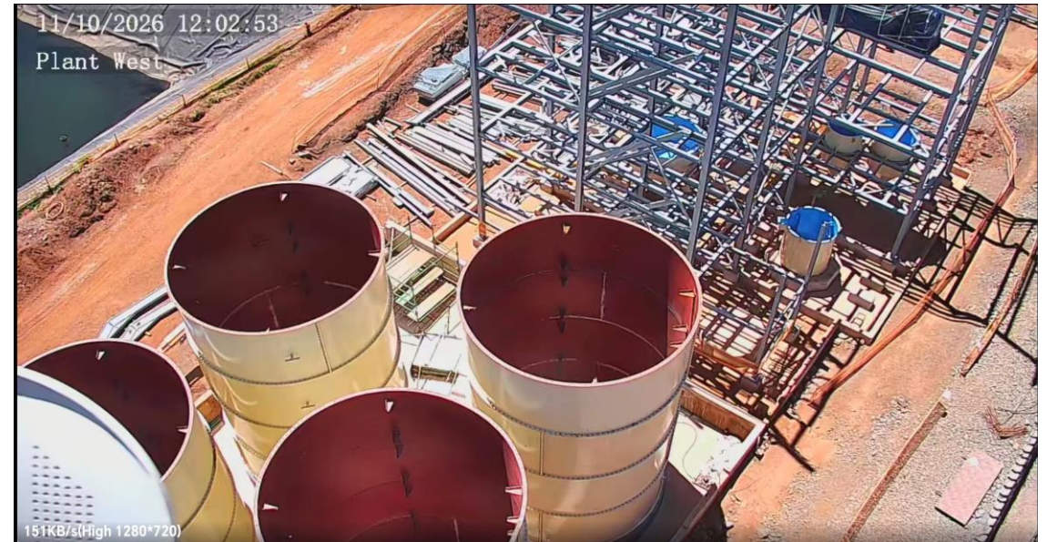
CIL Tanks and Elution Circuit erected
