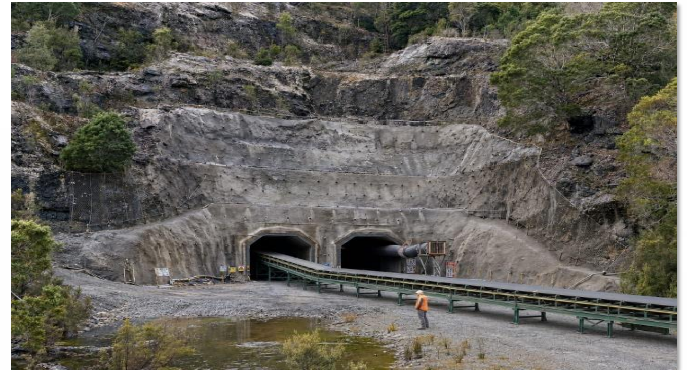
ILLUSTRATIVE TWIN-DECLINE PORTAL ARRANGEMENT
