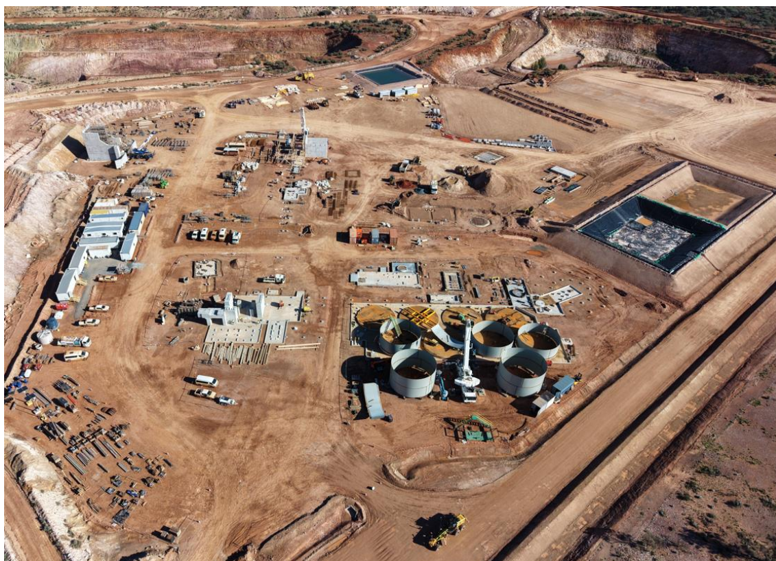
Figure 1 – Process Plant site construction progressing
