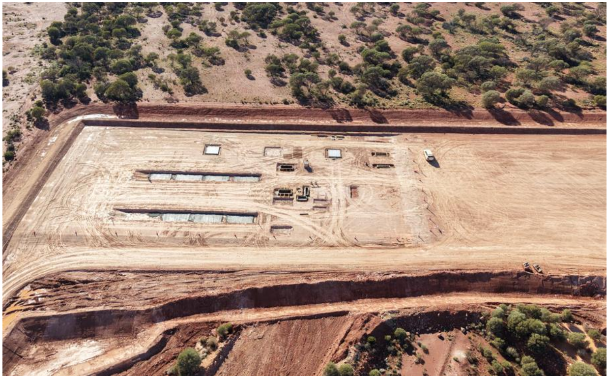
Figure 7 – Power station area – concrete commenced
