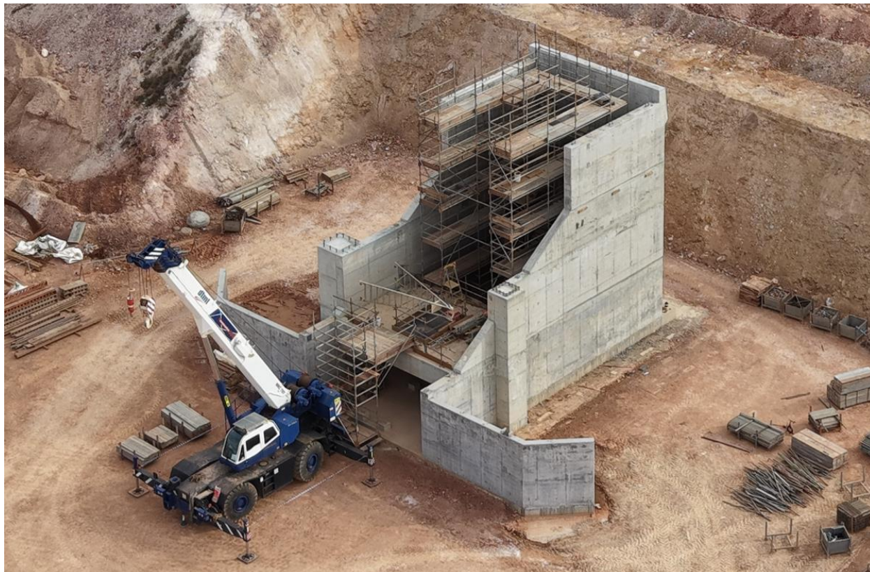
Figure 2 – Primary Crusher – final pour completed
