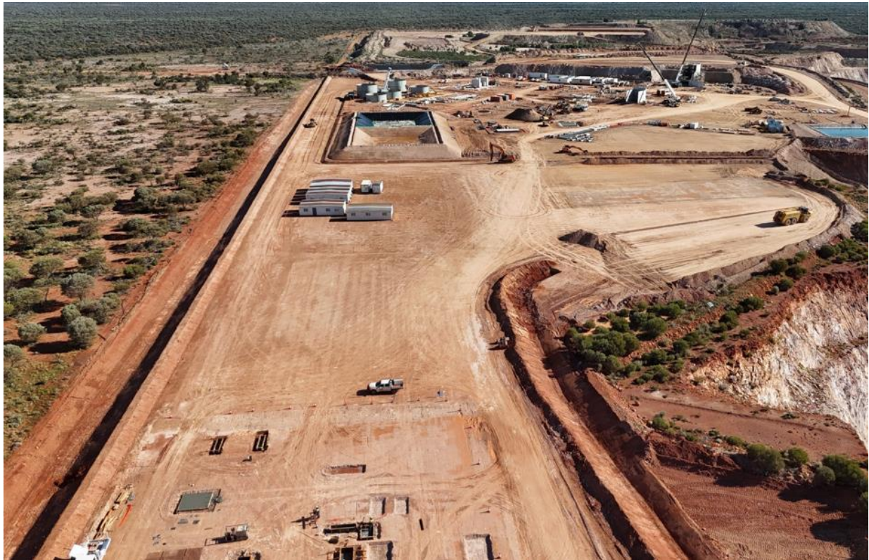
Figure 6 – NPI and Power Station areas – looking south towards the process plant
