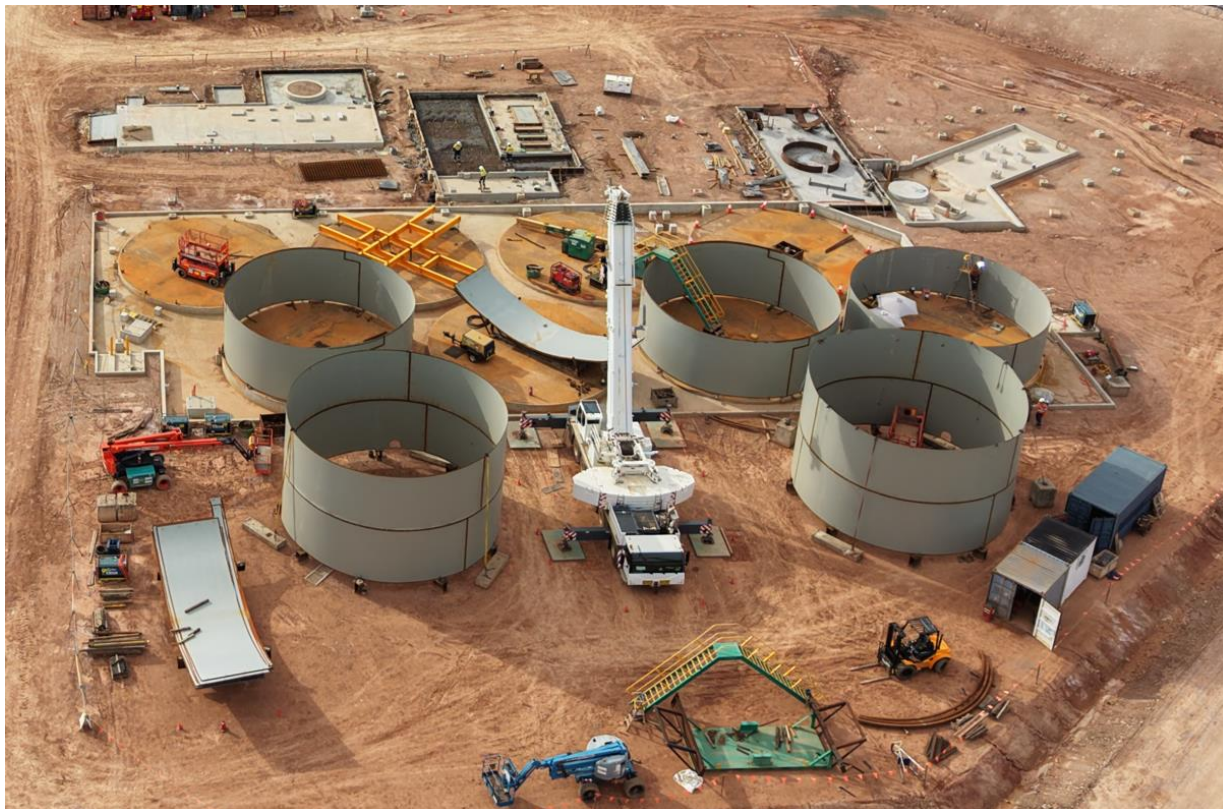
Figure 4 – CIL circuit – tank construction underway
