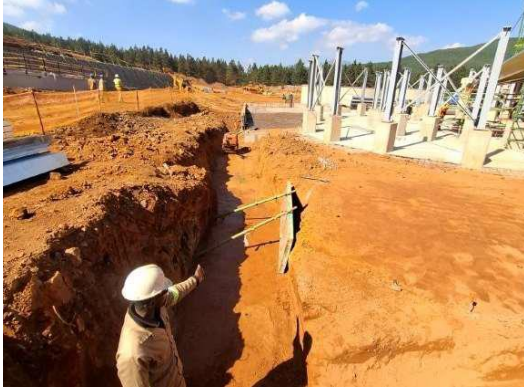
Excavation and Blinding release inspection of Thickener 600 bund wall.
