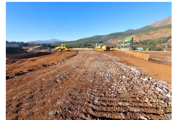
Road layer works being done on Road 1 at the southern end of the plant.
