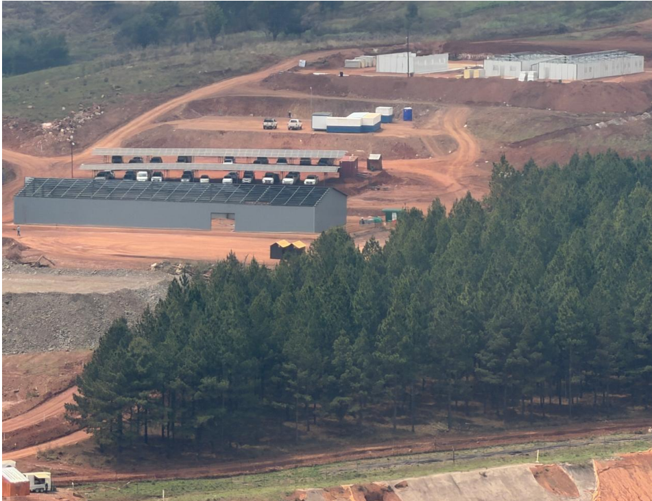
Management Offices, Solar Car Park, Goods shed
