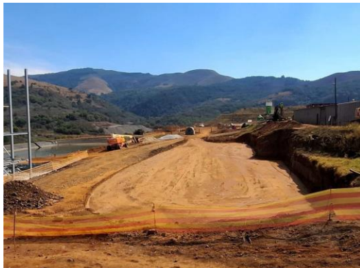
Area 800 Stabilenka installation completed and backfilled.
