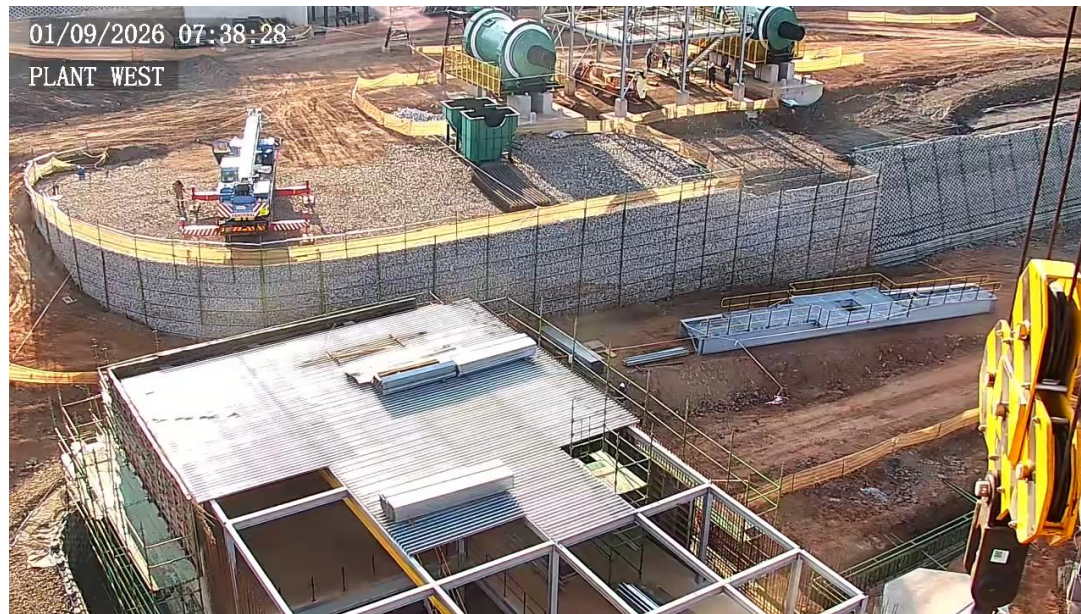
Gold Room Roof – under construction
