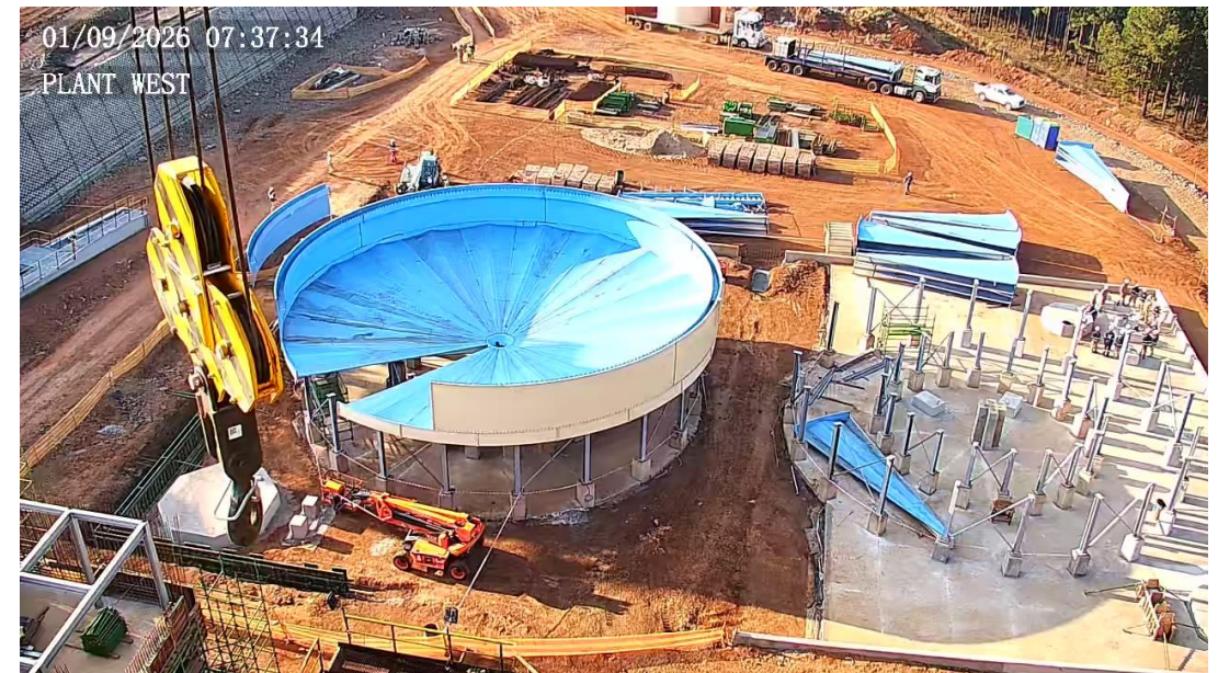
Thickener Tanks being constructed
