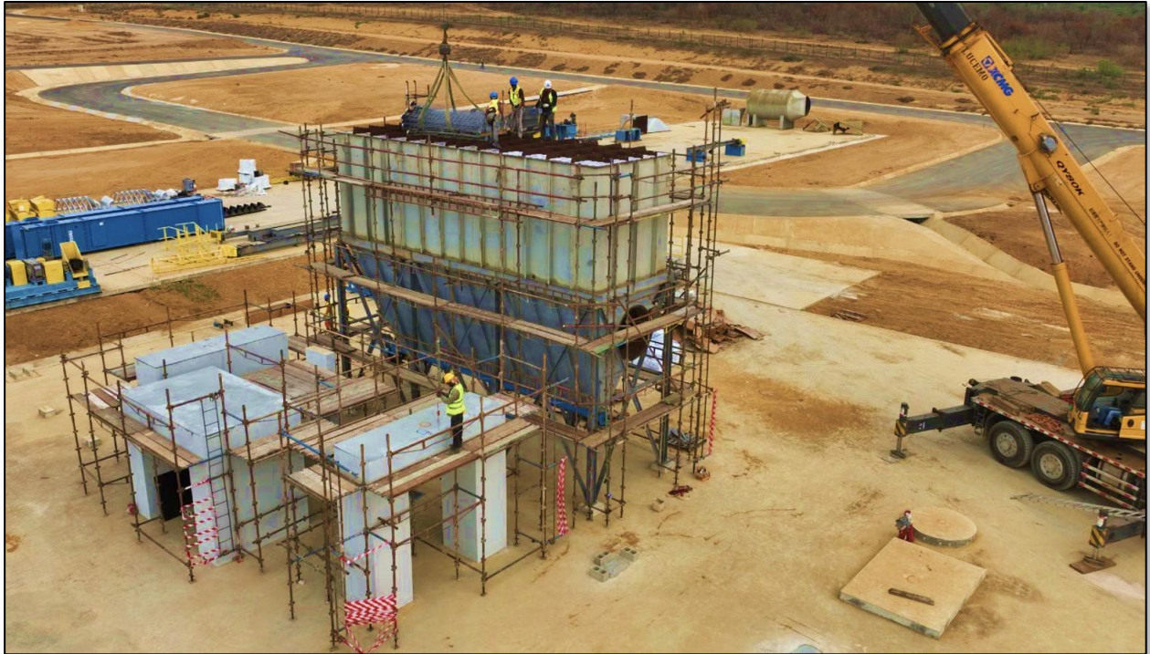
Figure 2 - Construction progress at the Cabinda Phosphate Plant, with installation works advancing on the main process infrastructure ahead of planned commissioning in 2027.
