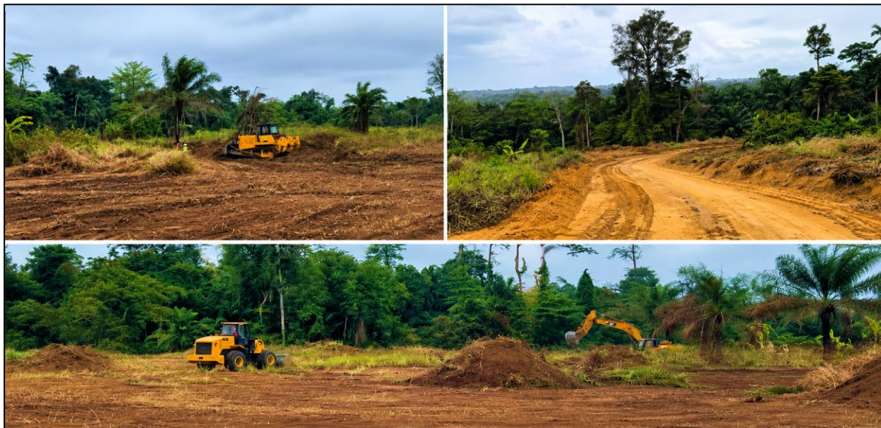
Figure 1 – Access-road clearing and preparatory earthworks at Cacata.
