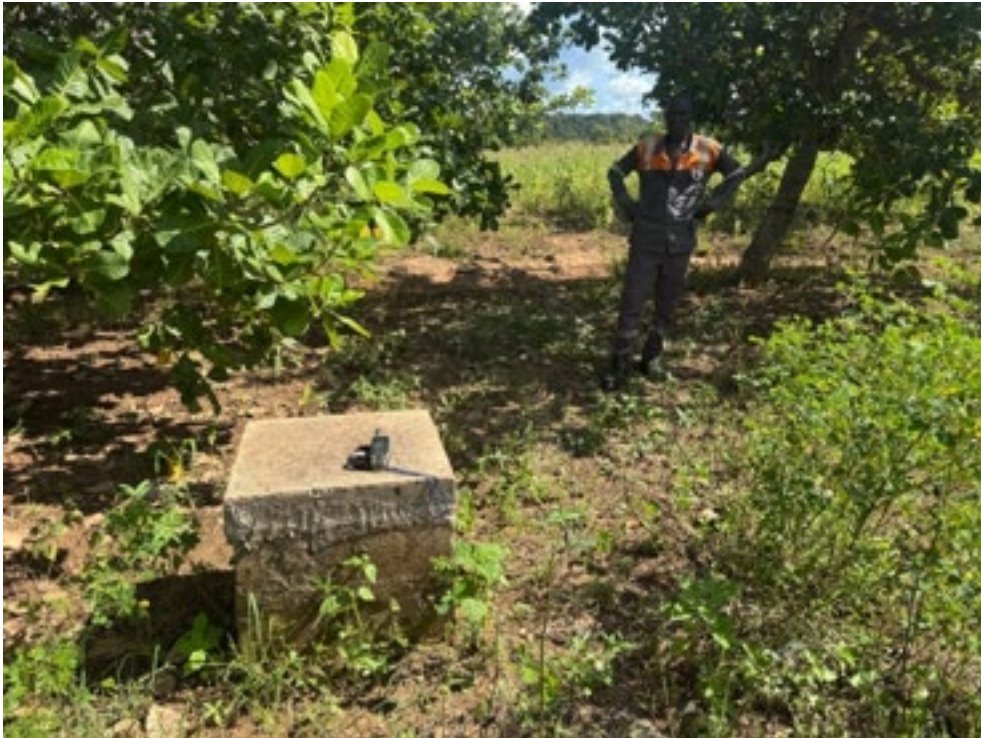
Figure 4: Drilling water borehole at Spodumene Hill still capped and appears to be in working condition
