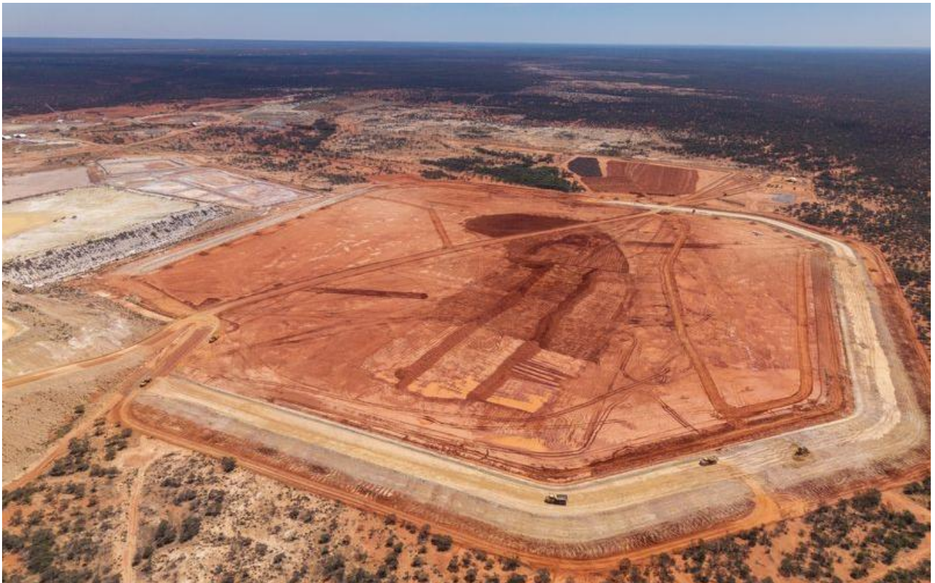
Figure 14 – Tailings Storage facility
