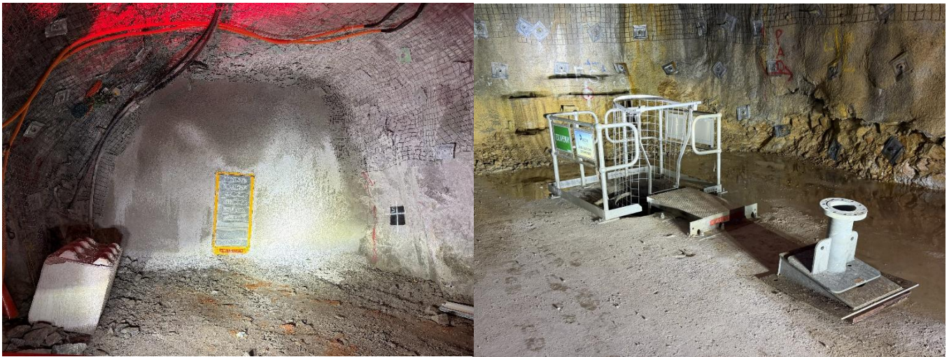
Figure 15 – United North core infrastructure advancing.
