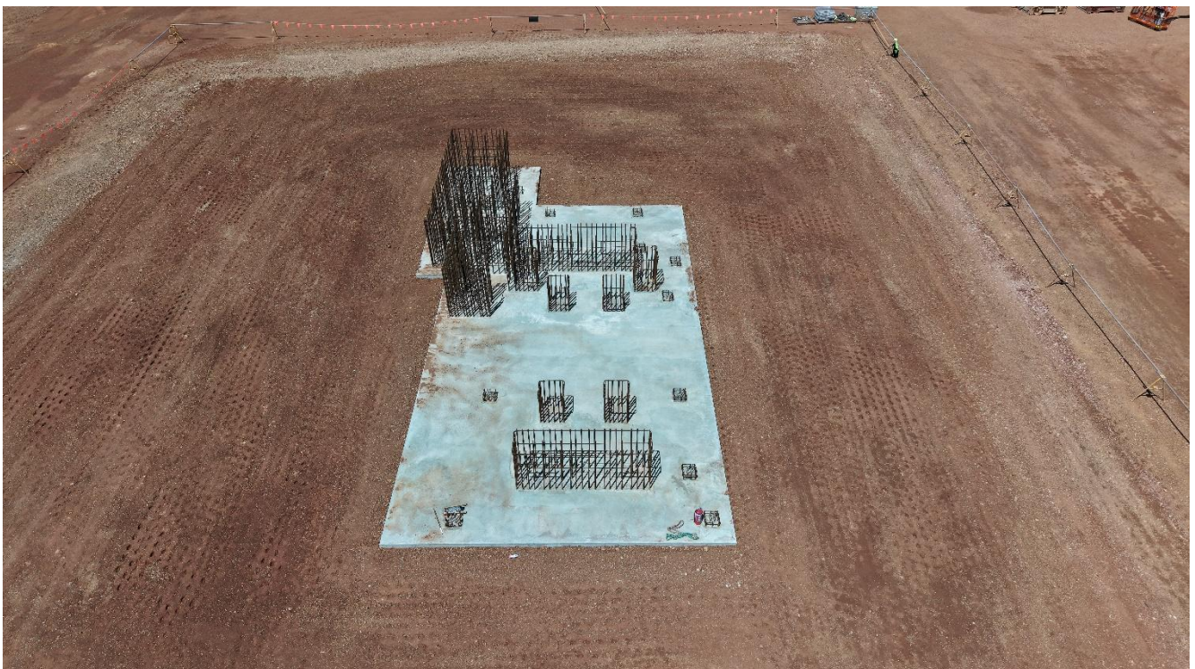
Figure 6 – Ball mill foundation completed reinforcement installation underway
