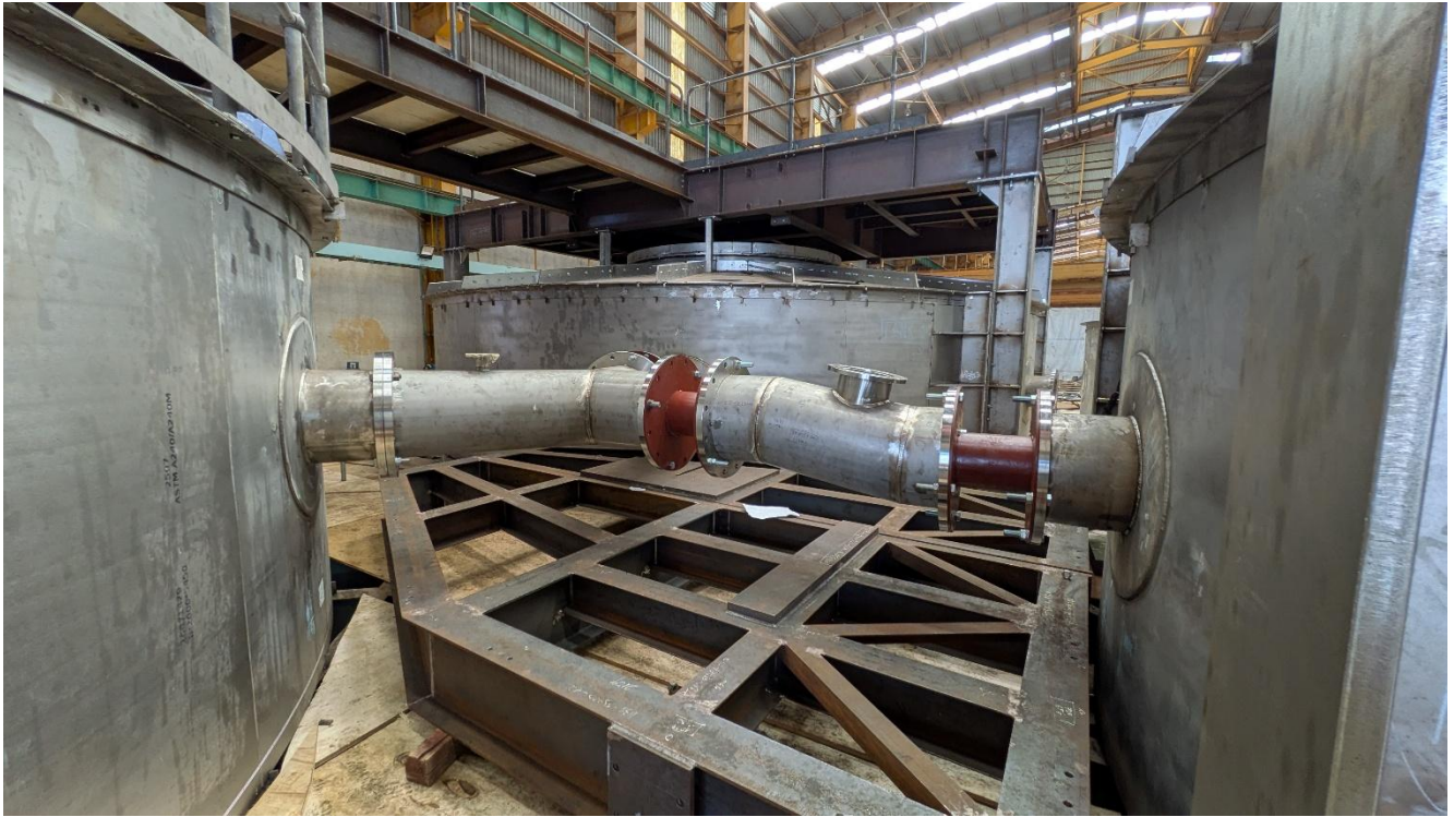
Figure 9 – Albion tanks fabrication & launder trial set up
