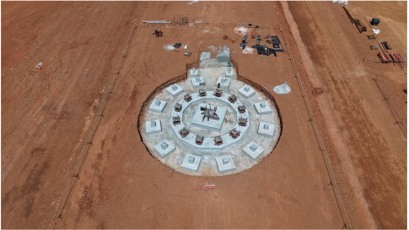
Figure 3 – Leach thickener concrete footings progressing
