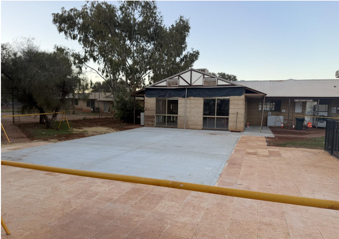
Figure 16 – Youanmi Wet Mess construction has commenced
