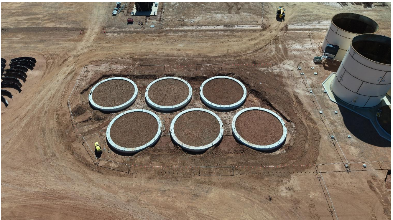
Figure 2 – Albion Tanks floors prepared
