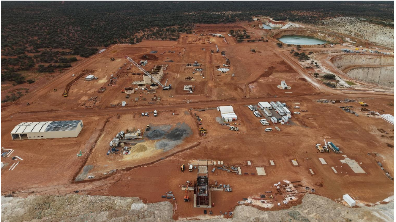
Figure 1 – Progress of construction on site – looking North
