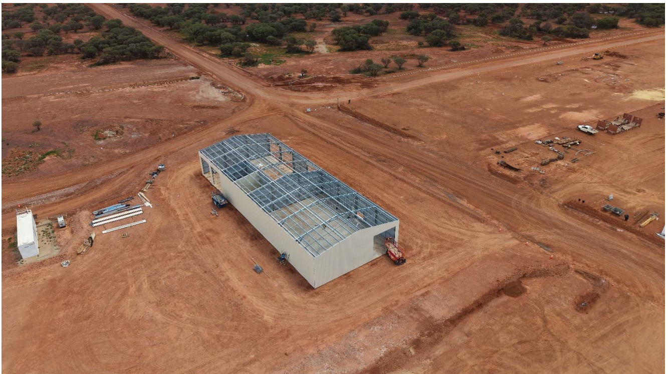
Figure 8 – Warehouse construction ongoing
