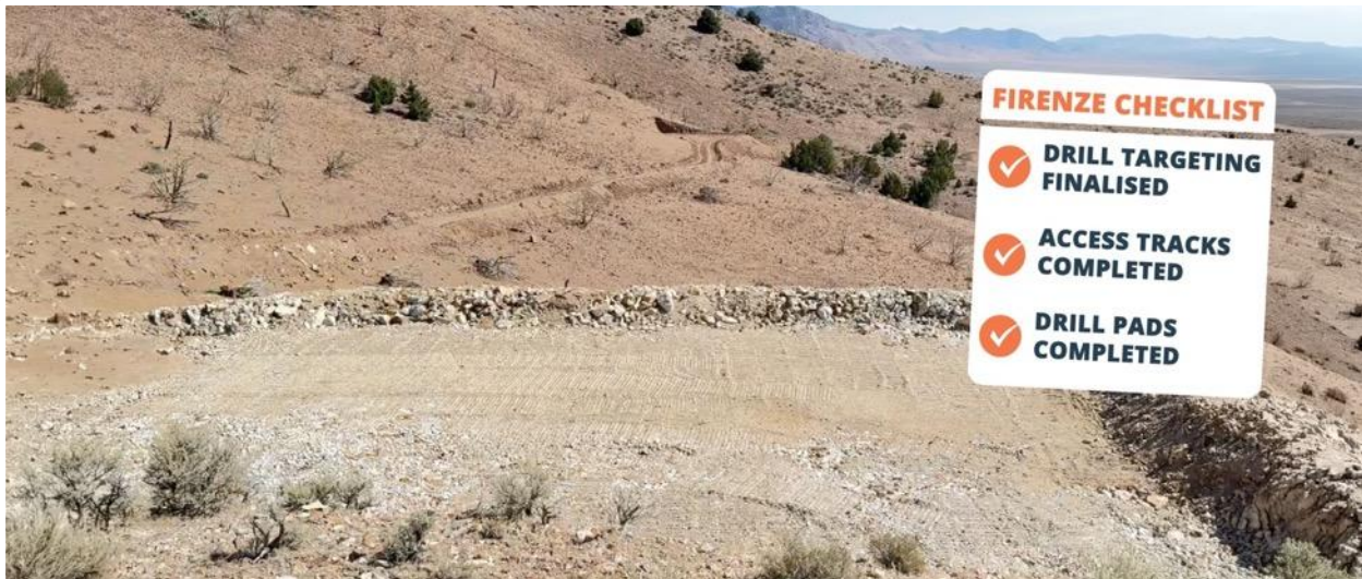
Figure 2. Completed access tracks and drill pads (August 2026)
