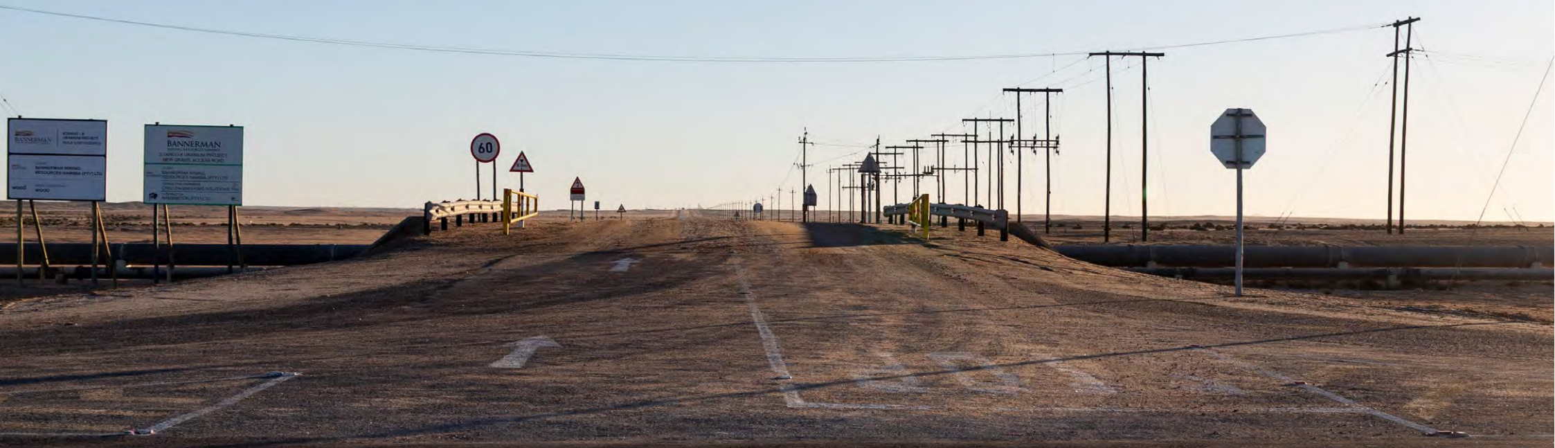
Left: Etango site access road at the C28 intersection Right: Secondary and tertiary crushing structure
