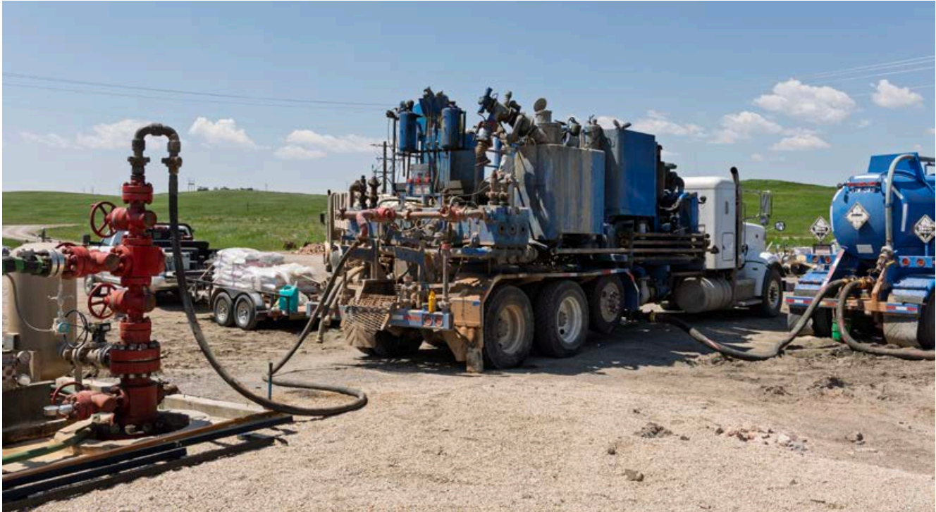
Figure 4-1: Mechanical integrity testing and acid simulation being performed on the deep disposal well
