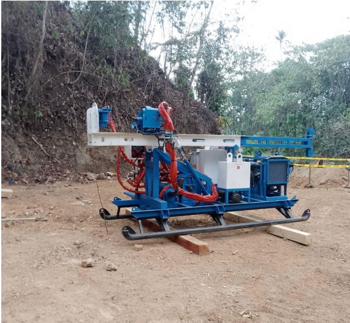
Figure 1: Drill rig mobilised to Pad 1, with the start of the Weioko Ridgeline seen in the background
