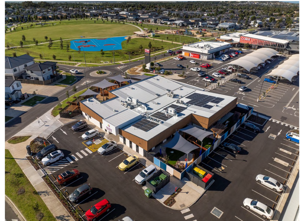
Newly acquired centre in Craigieburn, Victoria
