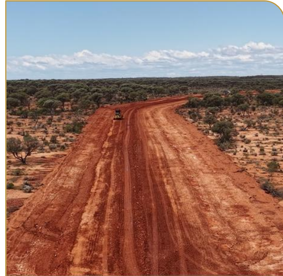
Mt Ida public road diversion commenced
