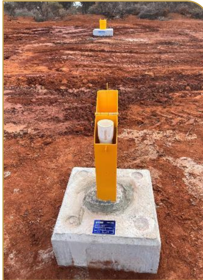
Production bore background and monitoring bore foreground
