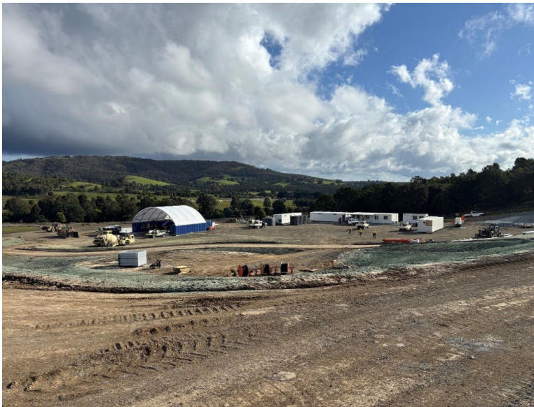
Figure 4. Site infrastructure area with workshop and site offices, August 2026.
