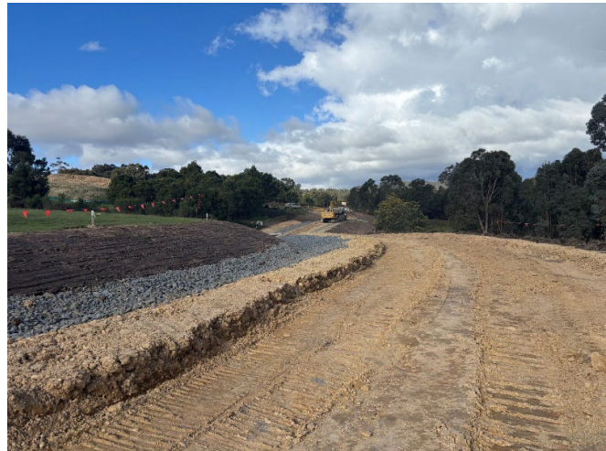
Figure 2. Main access road construction and infrastructure pad, August 2026.
