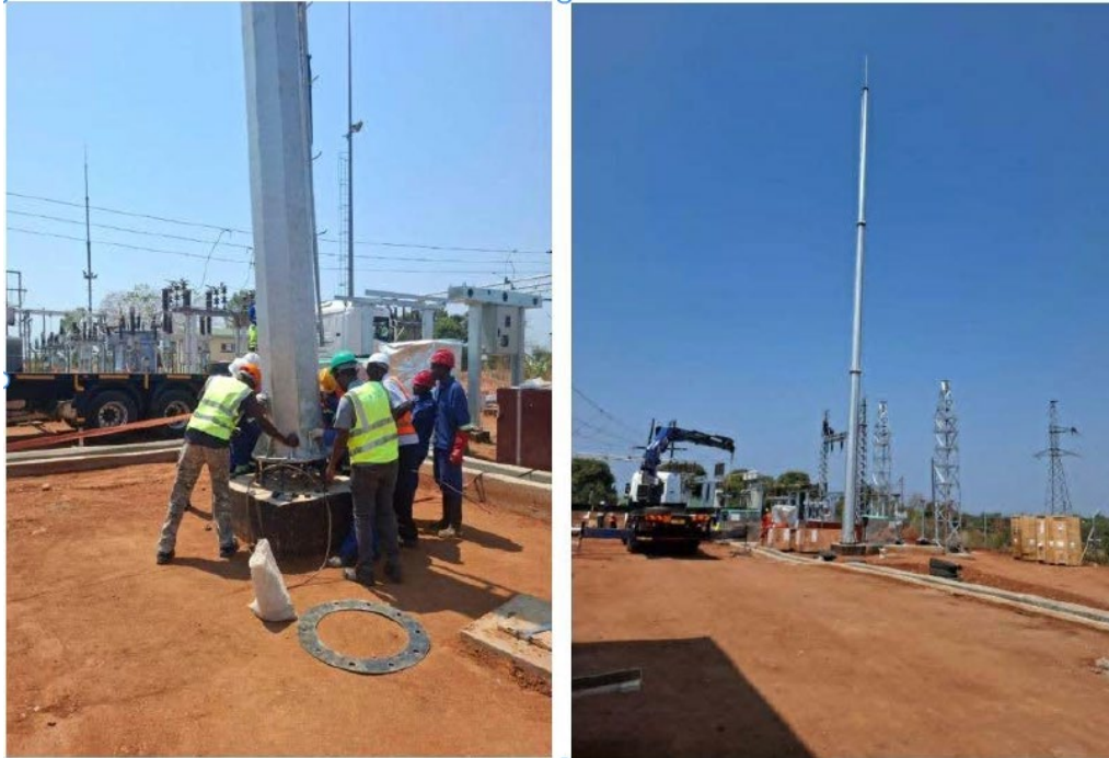
Figures 2 and 3: Grid Connection works
