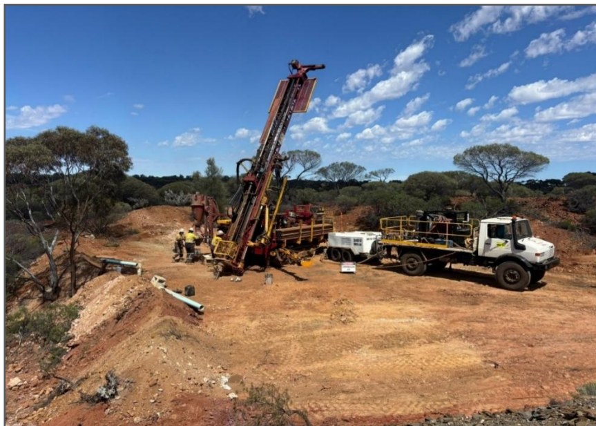
Figure 1: Drill rig on the first hole at Gulls Blow Prospect.
