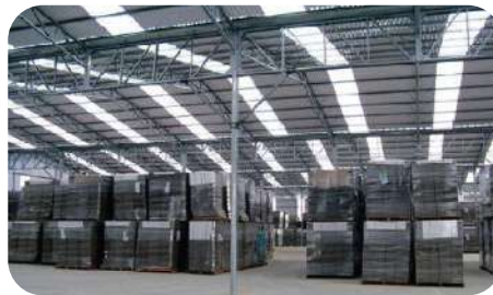
Transparent roof project to reduce lighting usage
