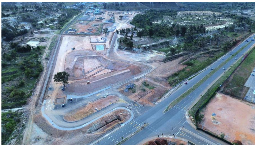
IMAGE 3: COMPLETED HAULAGE ROAD AND SITE ACCESS, WITH THE POLLUTION CONTROL DAM UNDER CONSTRUCTION
