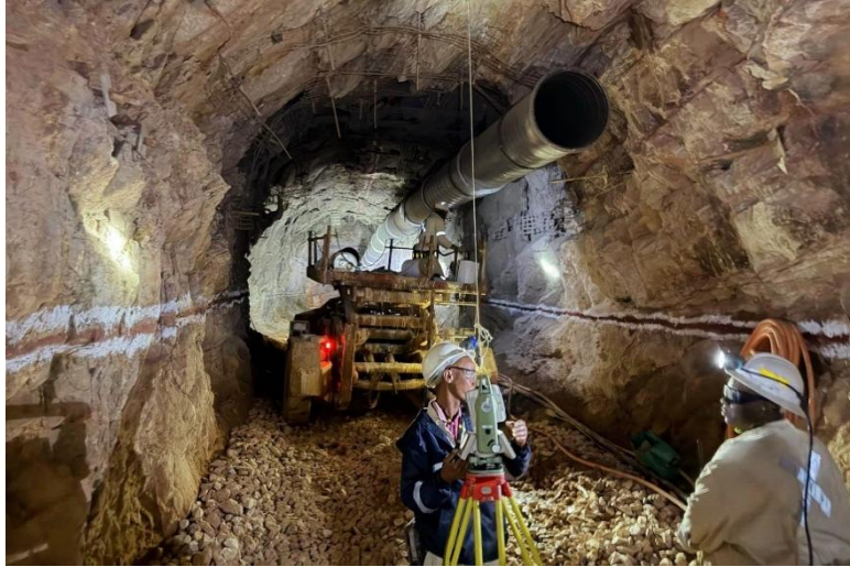
IMAGE 2: DEVELOPMENT DRILLING AND SURVEY AT AN UNDERGROUND FACE AT QALA SHALLOWS
