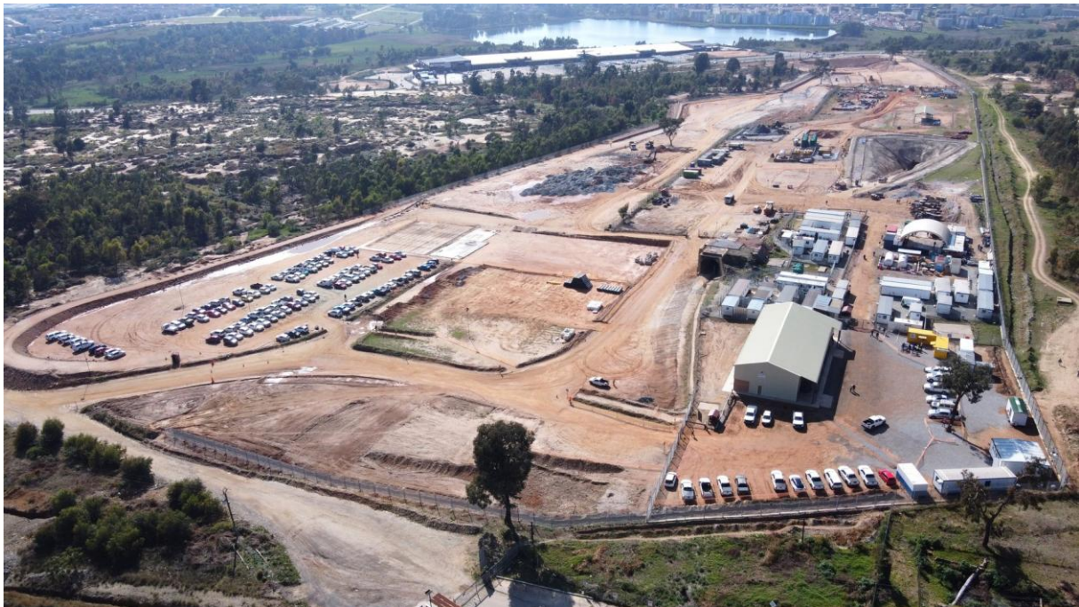
MAGE 1: AERIAL VIEW OF QALA SHALLOWS SHOWING THE DECLINE PORTAL, WORKSHOP, SITE OFFICES AND SURFACE INFRASTRUCTURE WORKS
