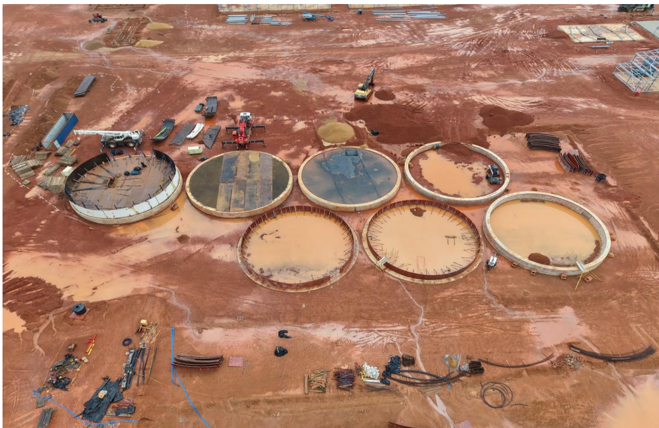
Photo 3: CIL Tank Erection in Progress
