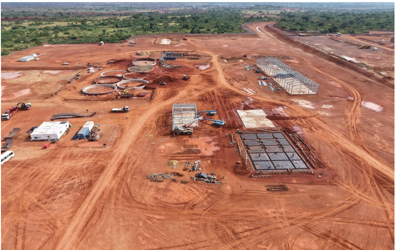
Photo 2: Process Plant – Bulk Earthworks Complete, Foundations in Preparation
