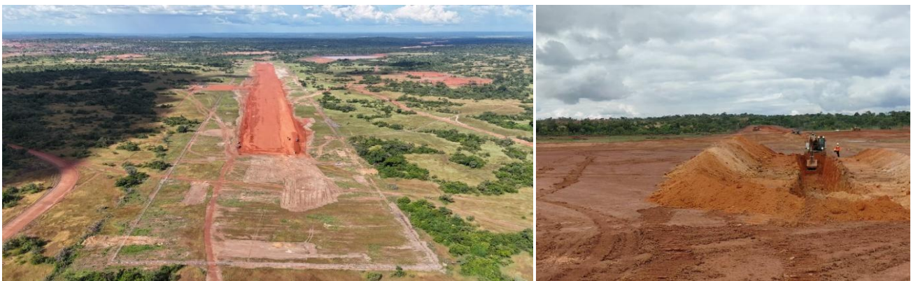
Photos 5 & 6: Airstrip Nearing Completion, TSF Western Embankment Construction in Progress
