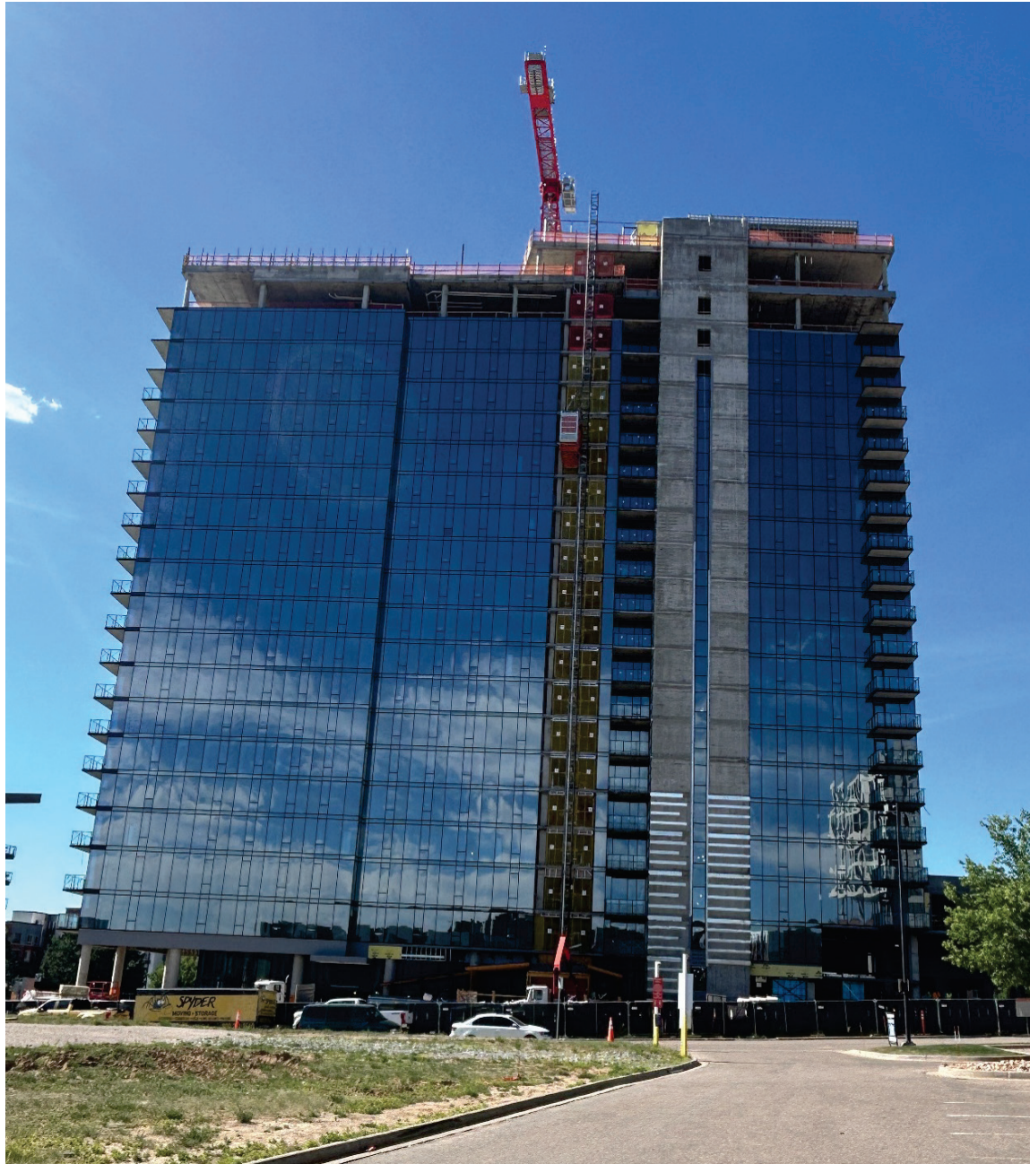
This 22-storey high-rise building - Bellview Station Block F – required 25,000 cubic yards of concrete that all included EdenCrete®Pz7. See Eden ASX Announcement 23 June 2025.
