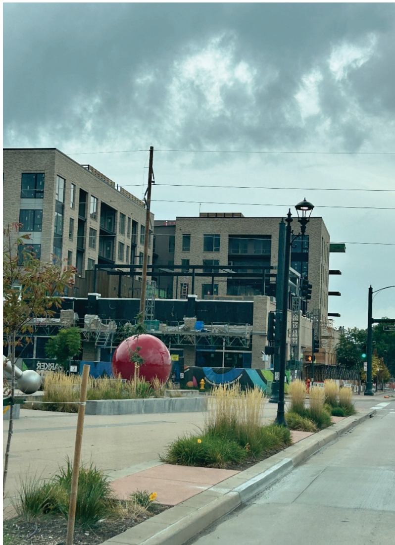
A building complex currently under construction in Denver area, Colorado using Pz7 concrete.
