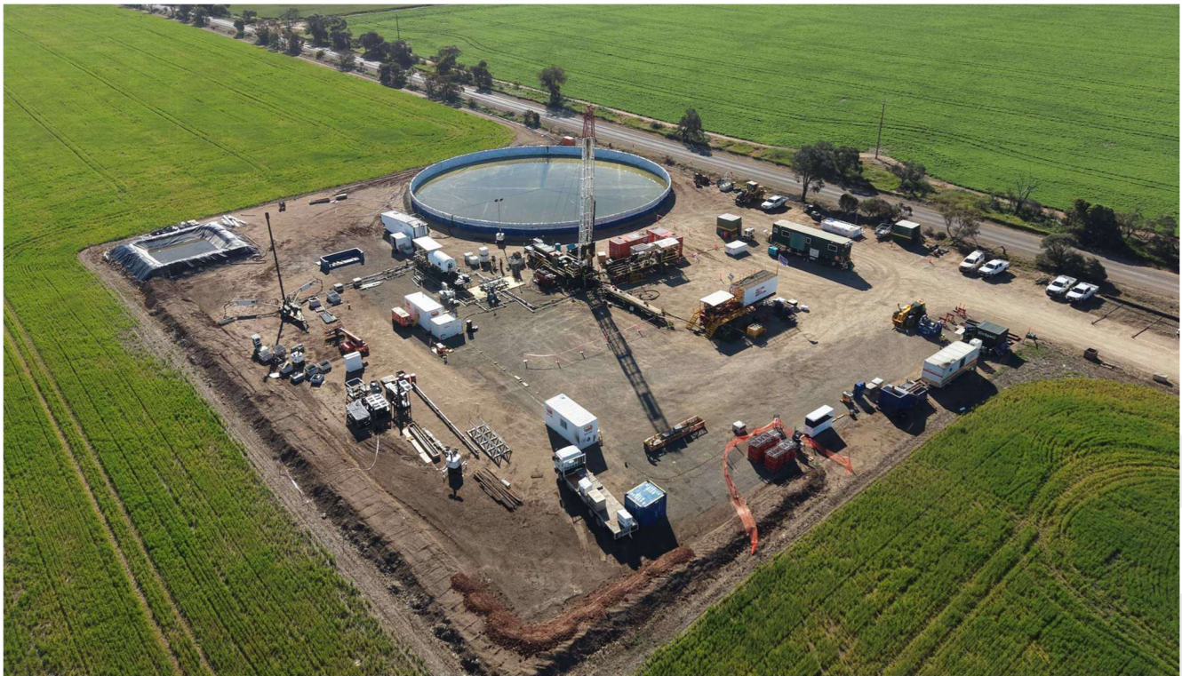
Ramsay 3 Wellsite during Phase 1 Helium Flow Testing
