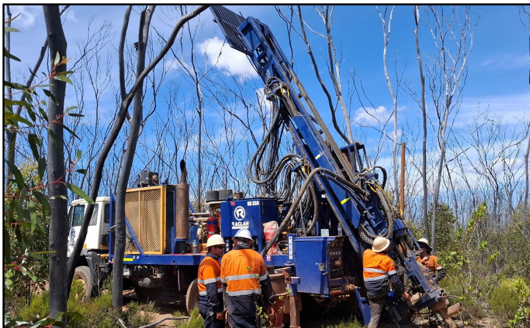
Figure 1: Commencement of drilling at the Norseman Project
