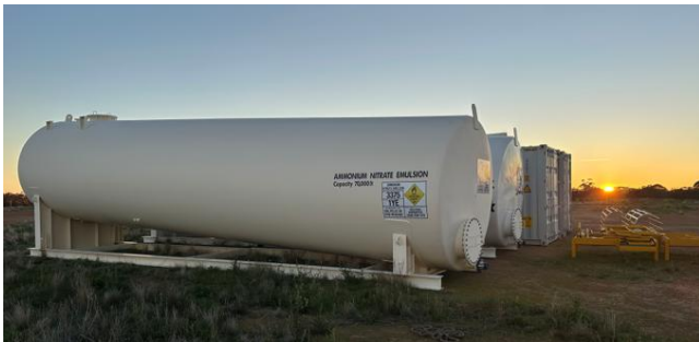
Fig 1. Tanks and dome for Brightstar mobilisation
