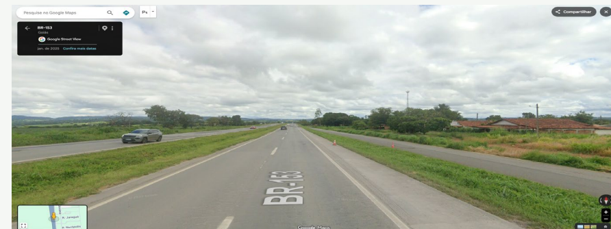
Condition of State Highway BR-153 (Belém–Brasília Highway), the main connection corridor to Goiânia.
