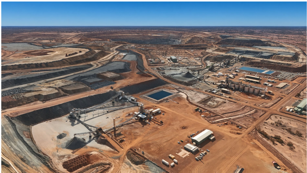
KEP (foreground) integrated into the broader Karlawinda Gold Project.
