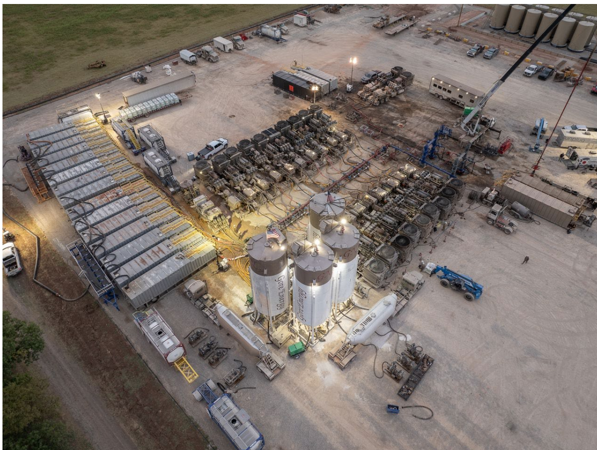
Stimulation Operations Underway on the Suttles Pad in Carter County, Oklahoma. Frac spread and sand silos in the centre and the tank battery visible in the top right of the photograph.
