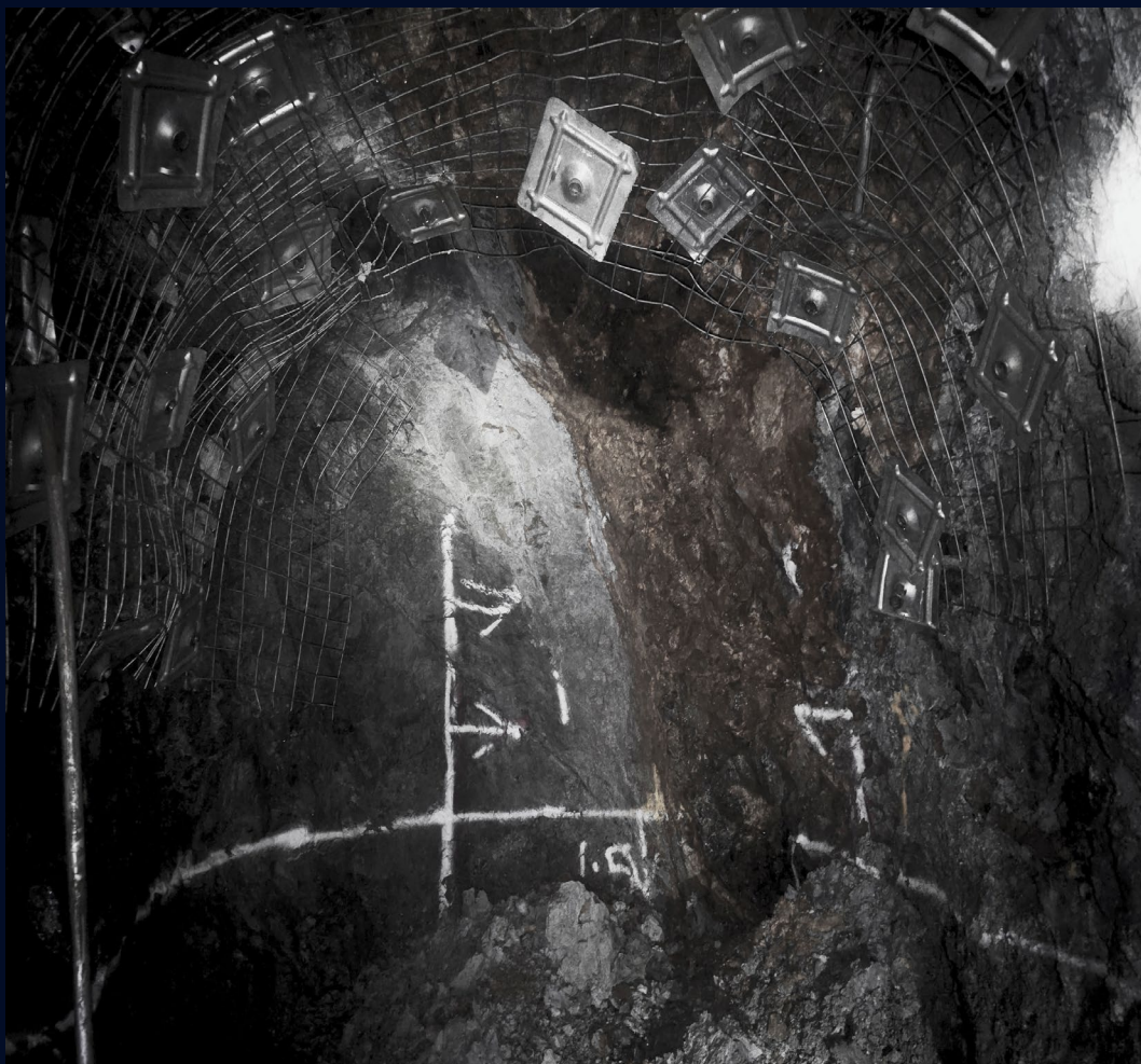
Ore drive development, 1560 Level — June 2026
