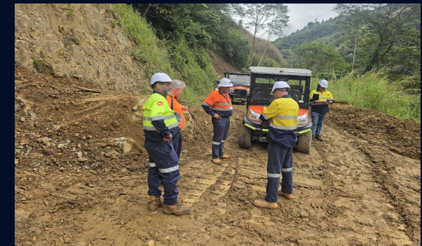
Lower portal area — June 2026
