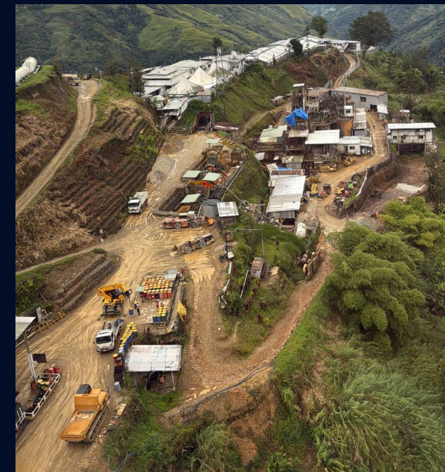
TGM processing facility — Tolukuma Gold Mine, June 2026
