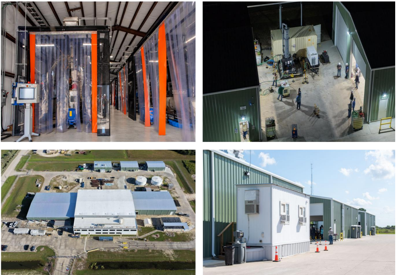
Figure 1: Gator Point Technology Campus, Texas, showing the FJH testing areas and multi-reactor operations, together with the recently repaired Area 140 roof and associated site infrastructure
