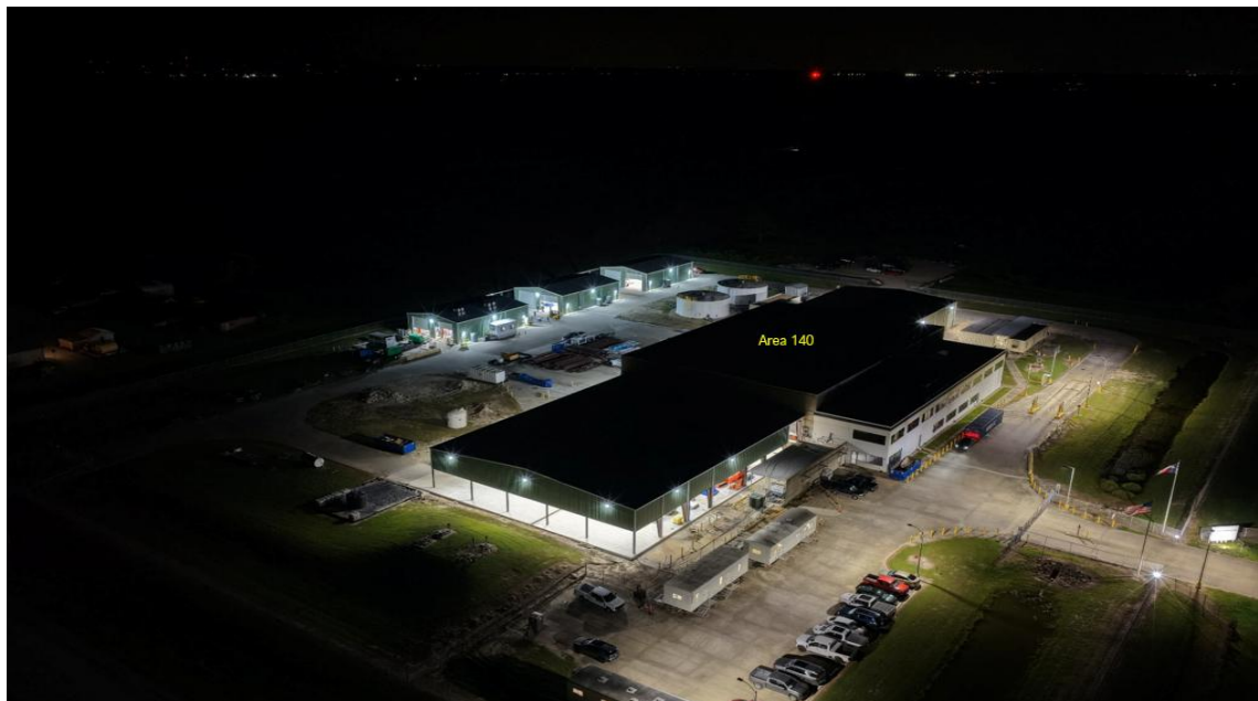
Figure 3: Gator Point Technology Campus during the Q3 multi-unit FJH campaign, with the newly restored Area 140 roof shown.
