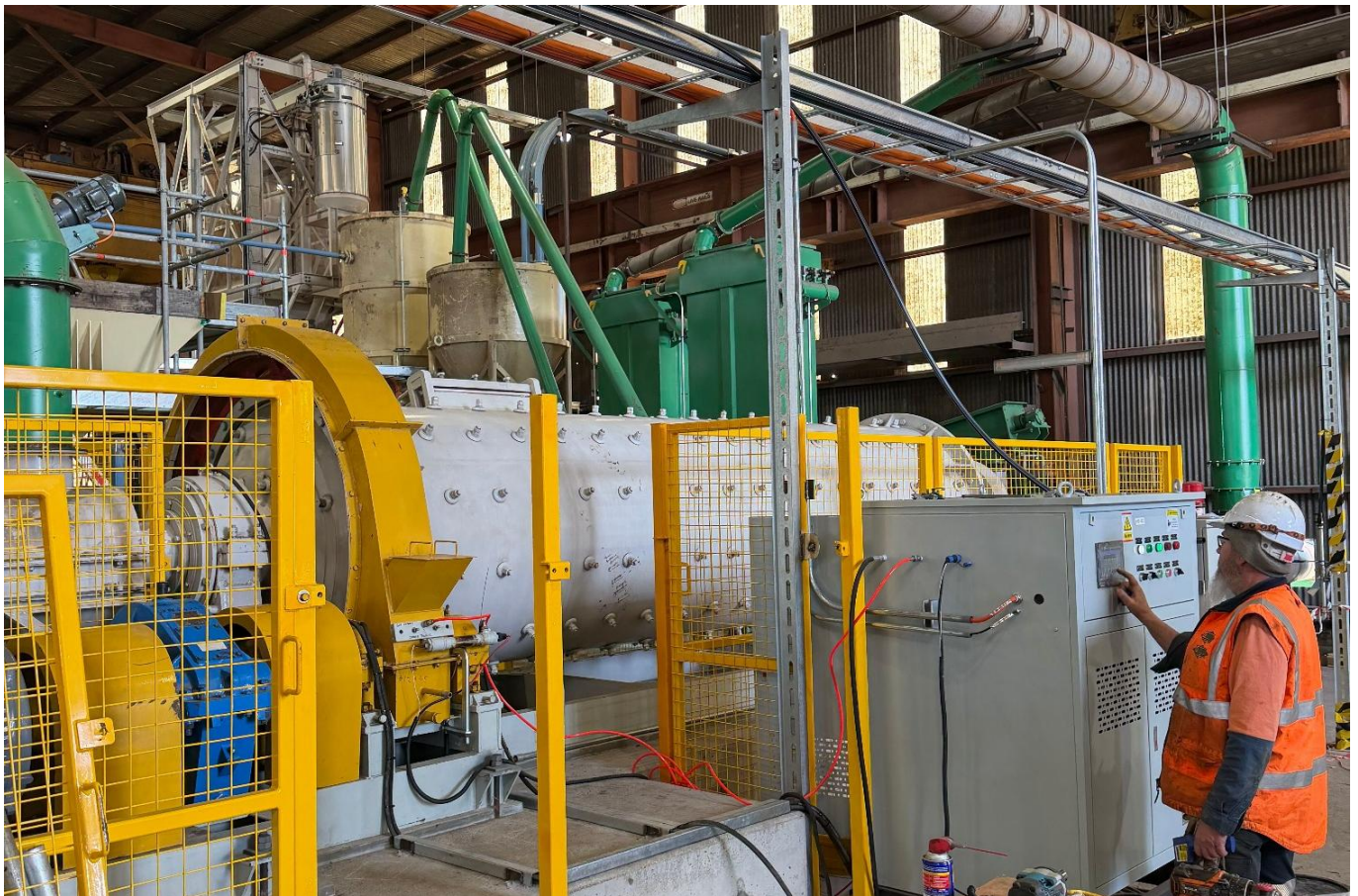
Figure 3: Commissioning and dry run of ball mill
