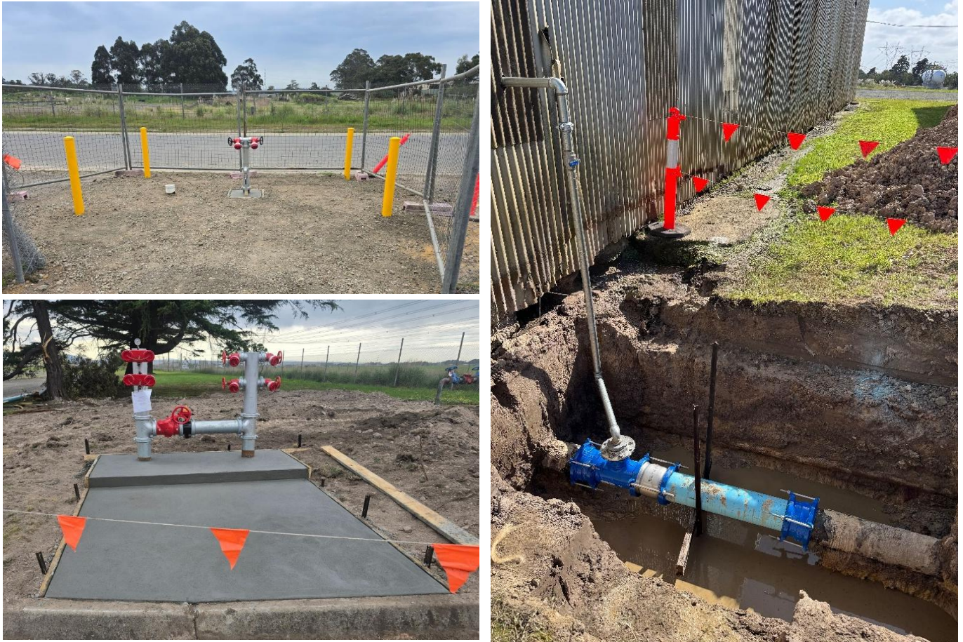
Figure 13: Progressive completion of fire protection system including quad booster system, isolation valves, and new hydrants
