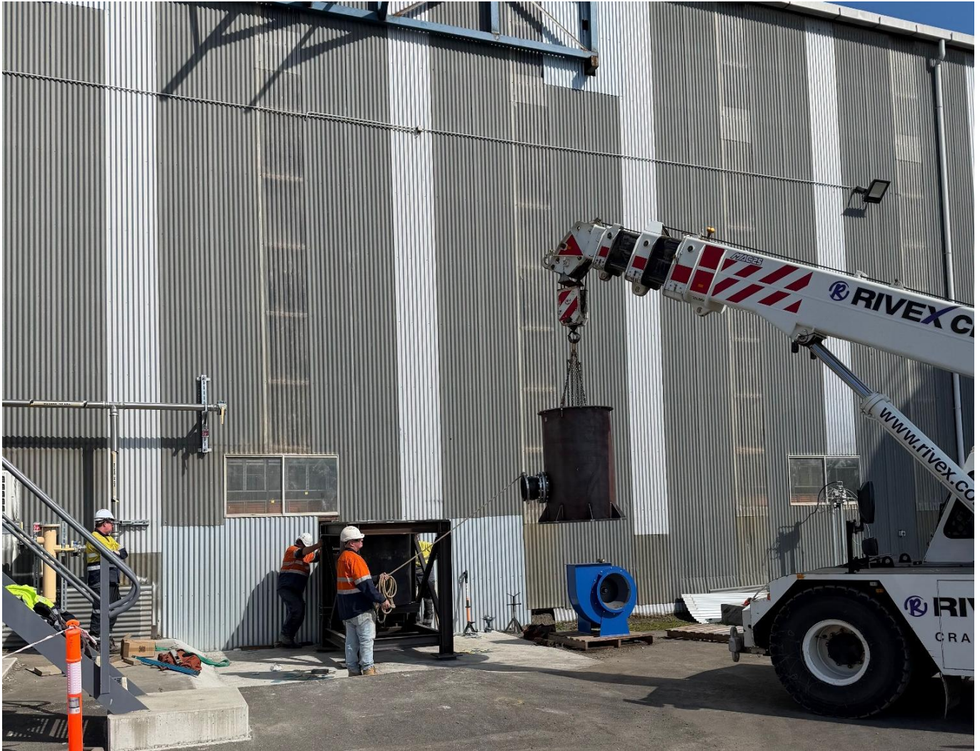
Figure 9: Exhaust Stack installation and lifting completed safely
