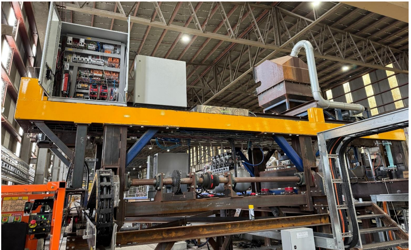
Figure 10: Automatic load shuttle terminations completed
