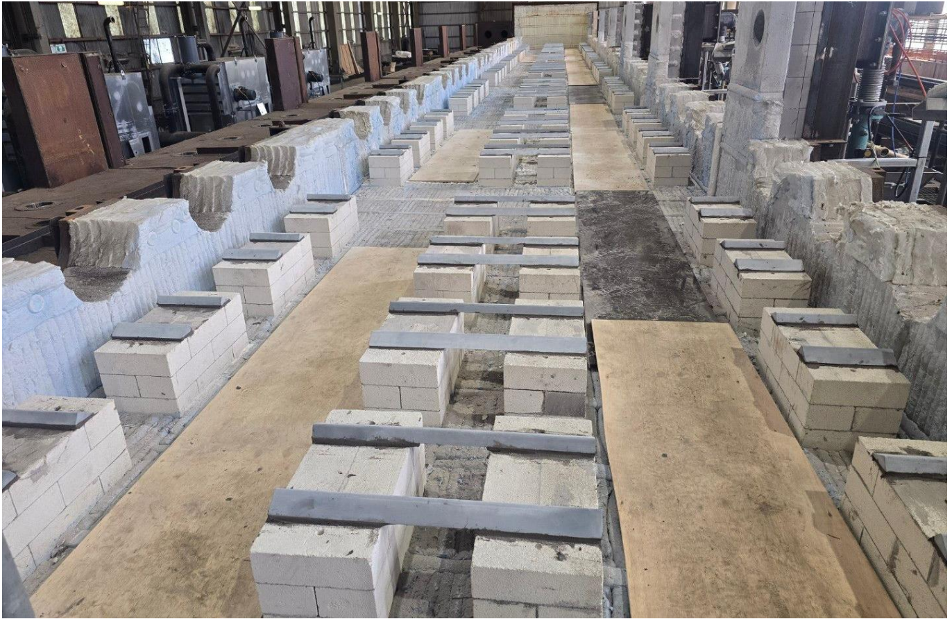
Figure 2: Retort pier installation complete
