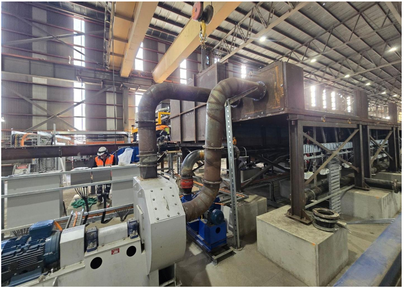
Figure 5: Reduction Furnace installation substantially complete with installation of ducting, fans, and piping
