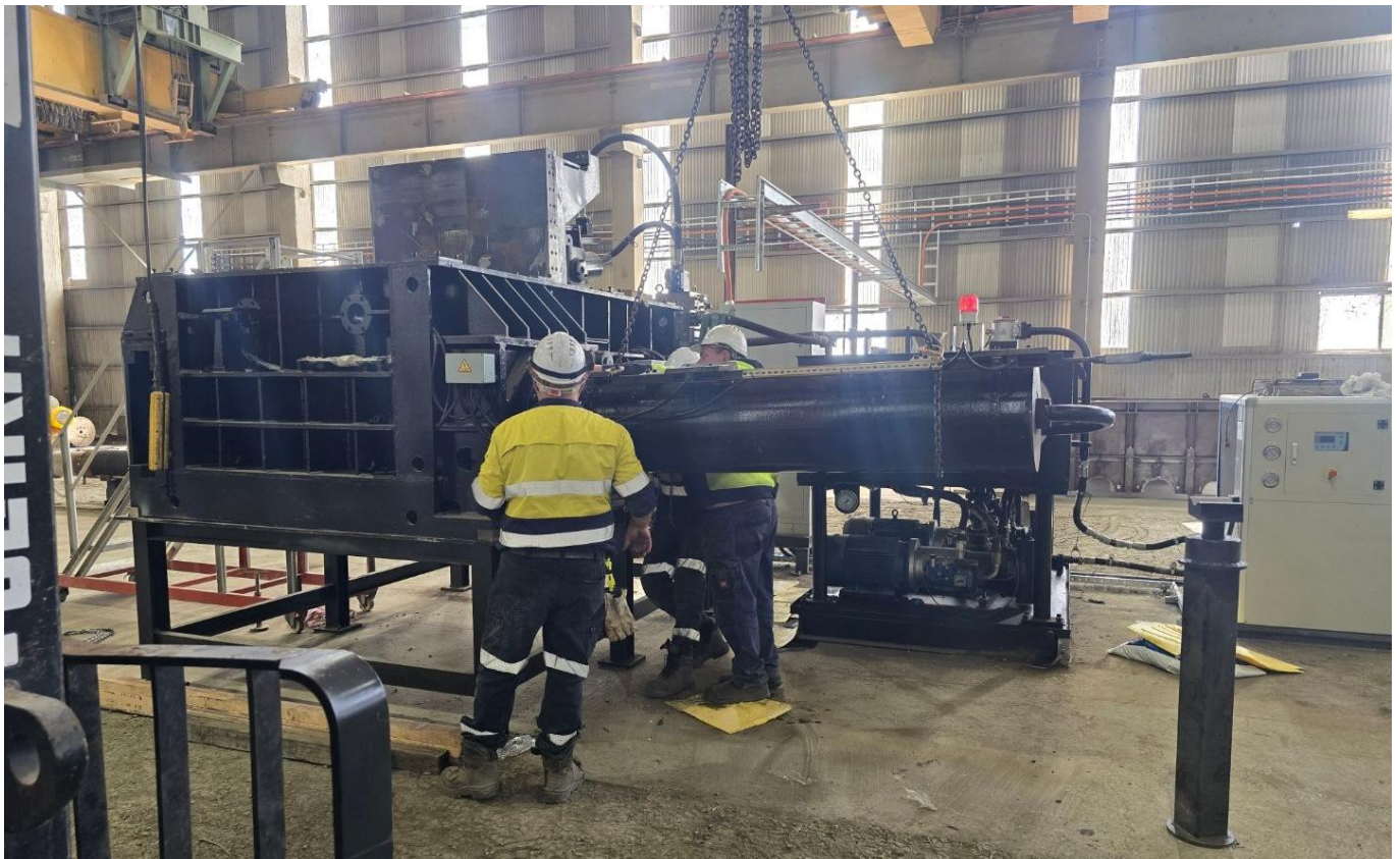
Figure 7: Crown Handling Baler installation
