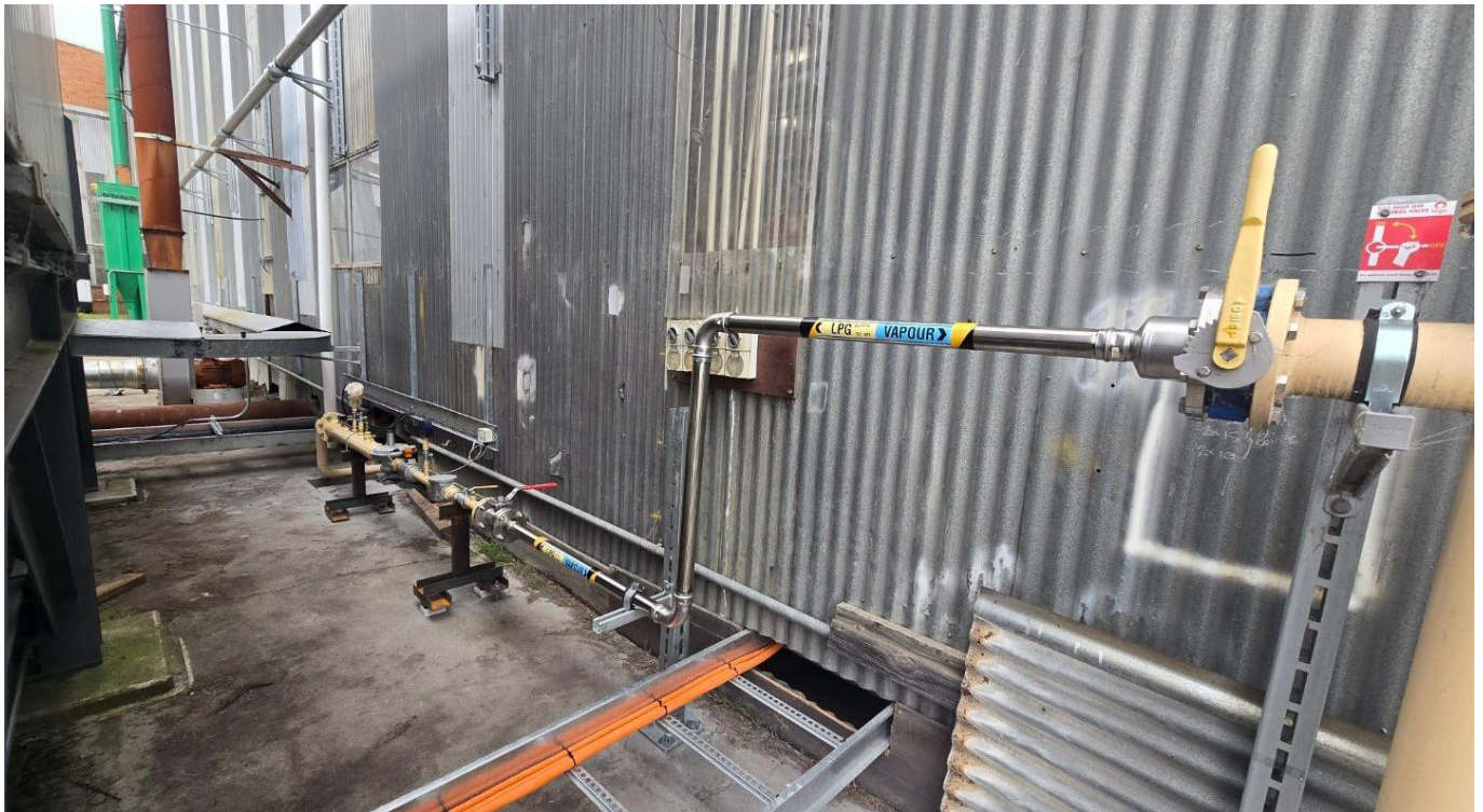
Figure 6: LPG supply infrastructure tie-in works completed by LPG vendor
