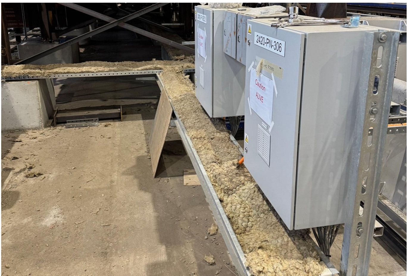
Figure 11: Cable tray insulation and protection progressing
