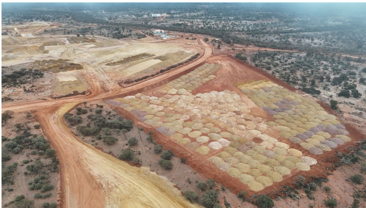
Figure 3: Ore stockpiling at the Redcastle Gold Project
