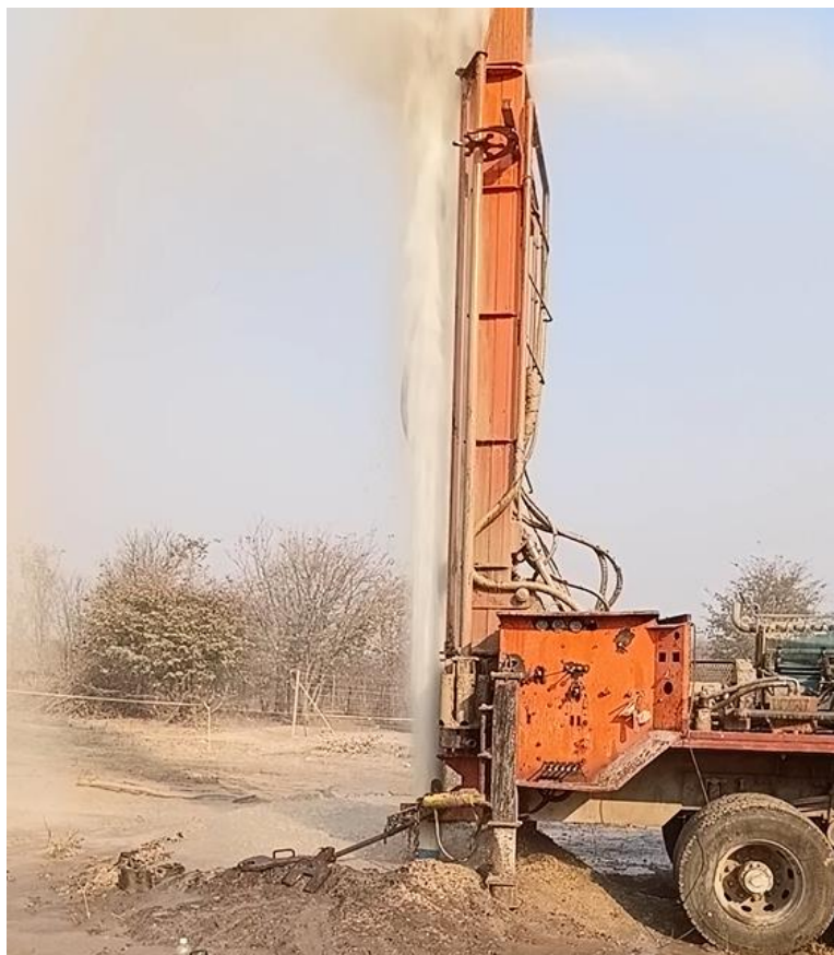
Figure 2: Water bore drilling, showing water under pressure escaping from the aquifer.
