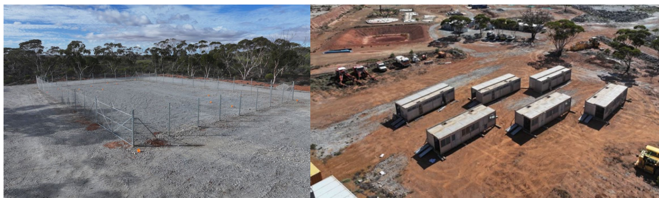
Photo 3 and 4: New magazine fencing and earthing and WIN dongas undergoing refurbishment
