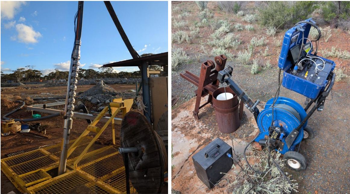
Photo 5 and 6: Dewatering pump being lowered into the shaft and Bore field investigations
