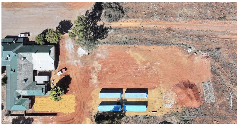
Photo 7: Rear of tavern, location of new camp install to incorporate all 10 donga blocks
