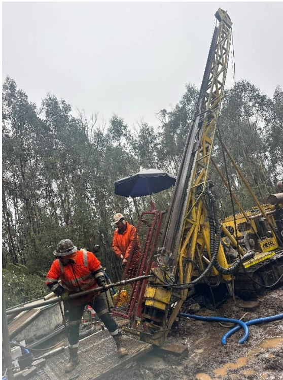
Figure 3: Drilling underway of 26SSDH004
