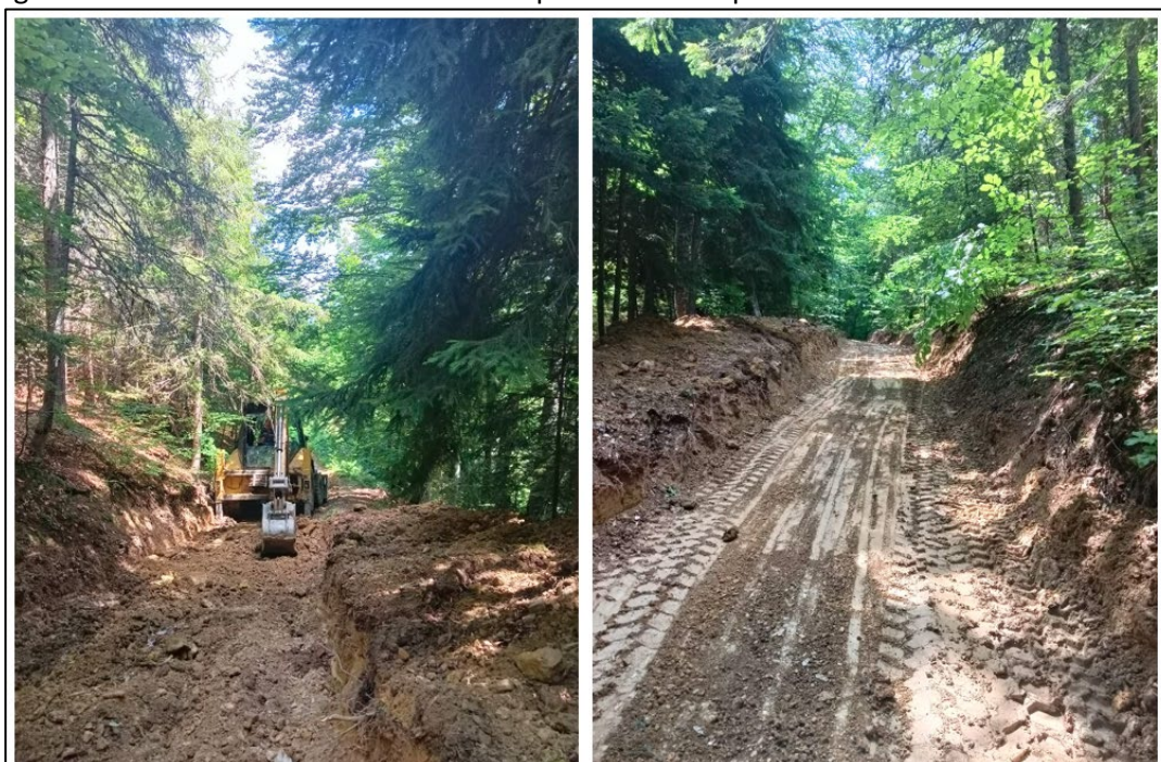
Figure 8: Monte Project, Pisonica Ag-Pb-Zn Prospect, photos of forest track repairs for drill site access
