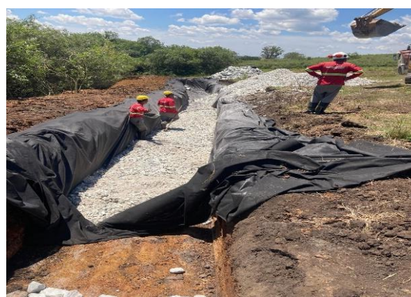
Image 4: Drainage to sump advancement
