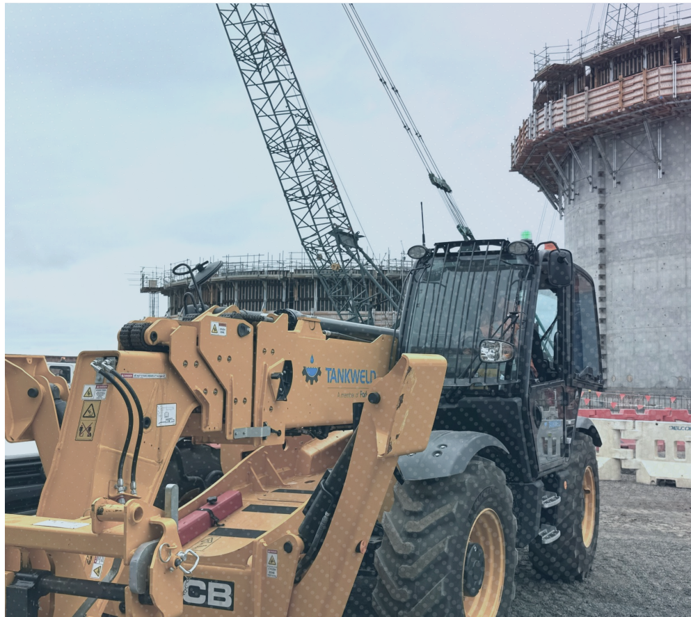
Parkway telehandler and operator performing SMP related construction activities for major water infrastructure project in Victoria.
