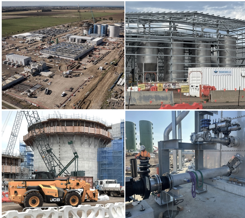
Key SMP scope for major resource recovery and reuse complex being successfully executed by Parkway.
