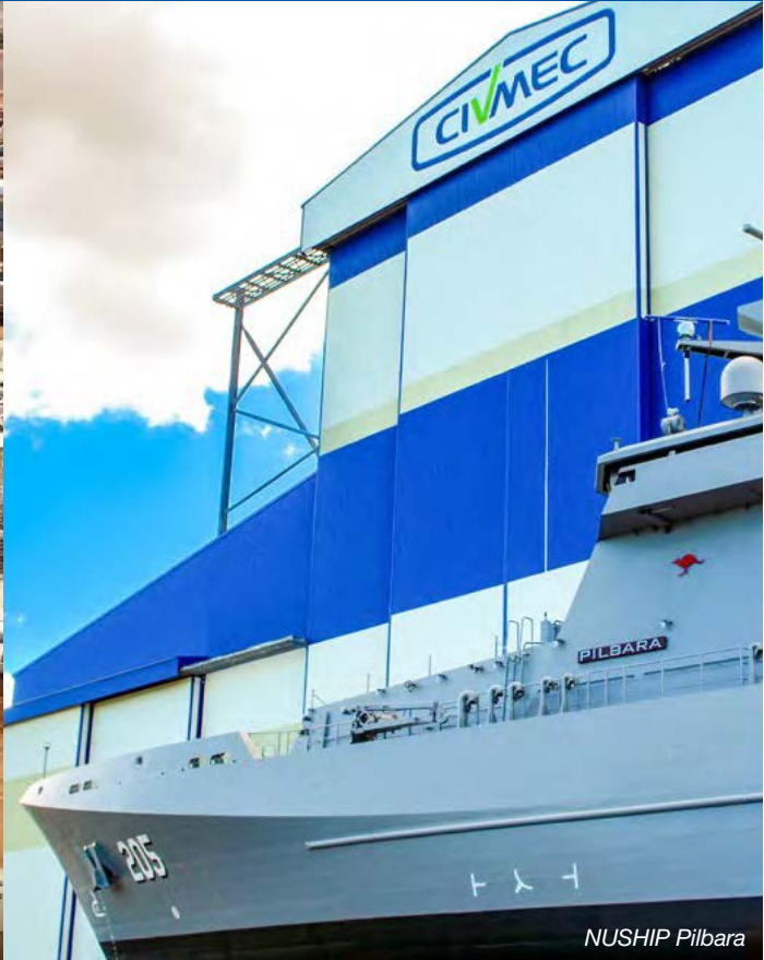
Eneabba Rare Earths Refinery
