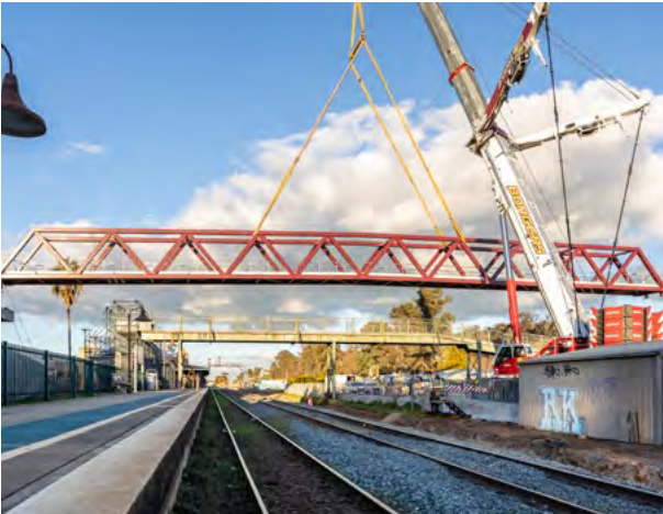
Albury to Illabo Footbridges
