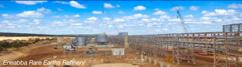
Eneabba Rare Earths Refinery
