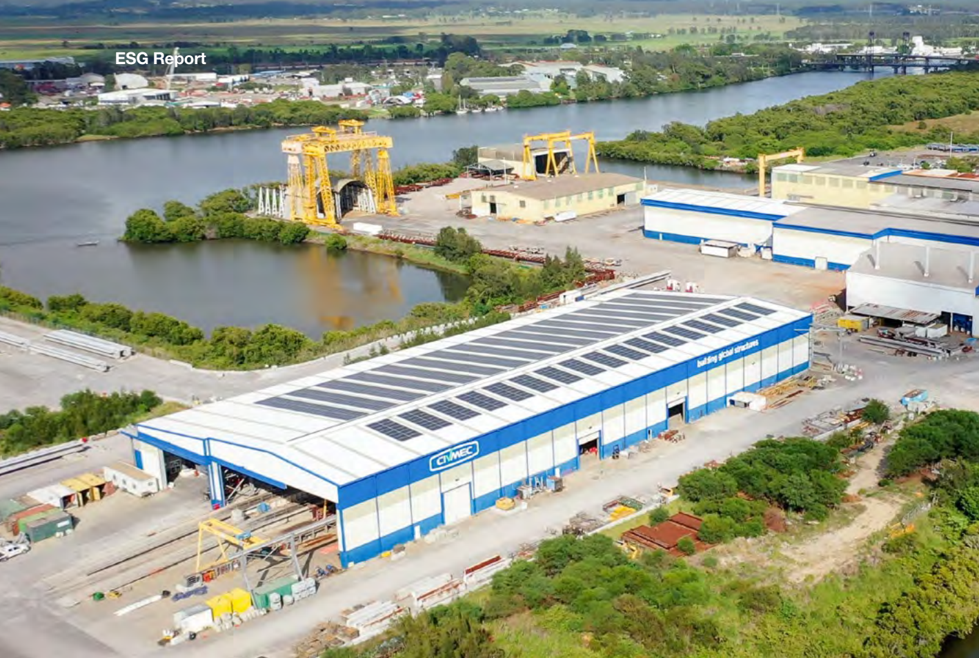
Solar PV infrastructure at Newcastle
