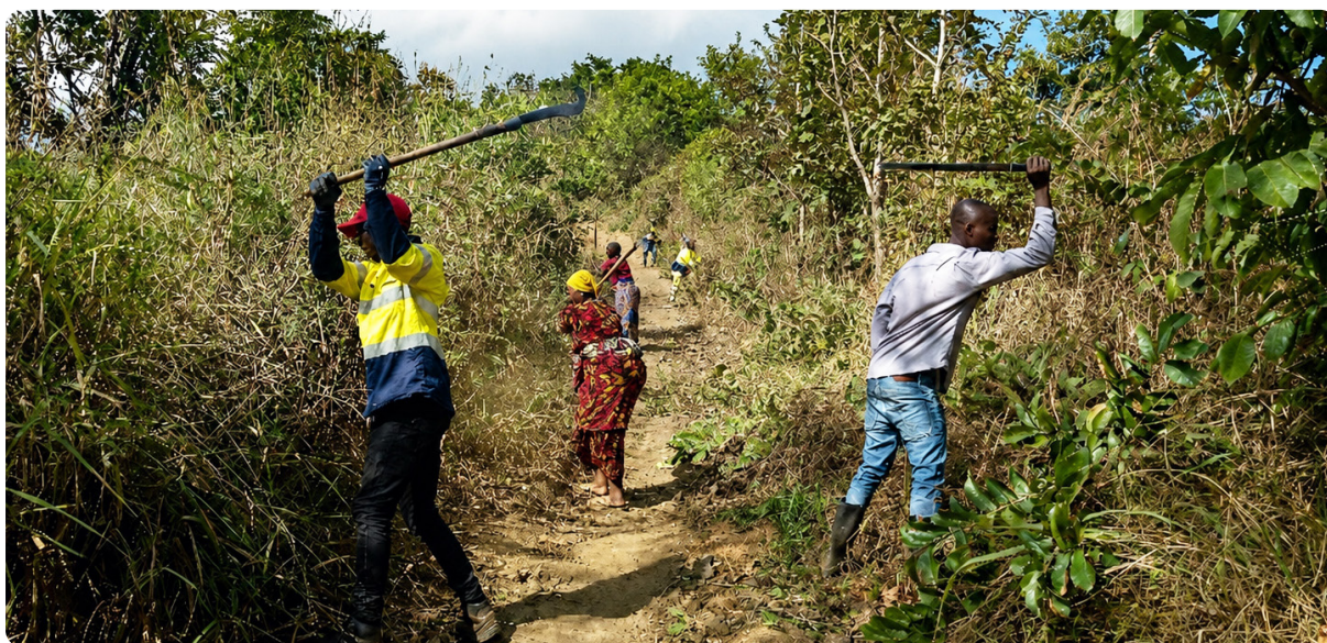
Figure 3: Kisewe Village Improving Community Access Tracks
