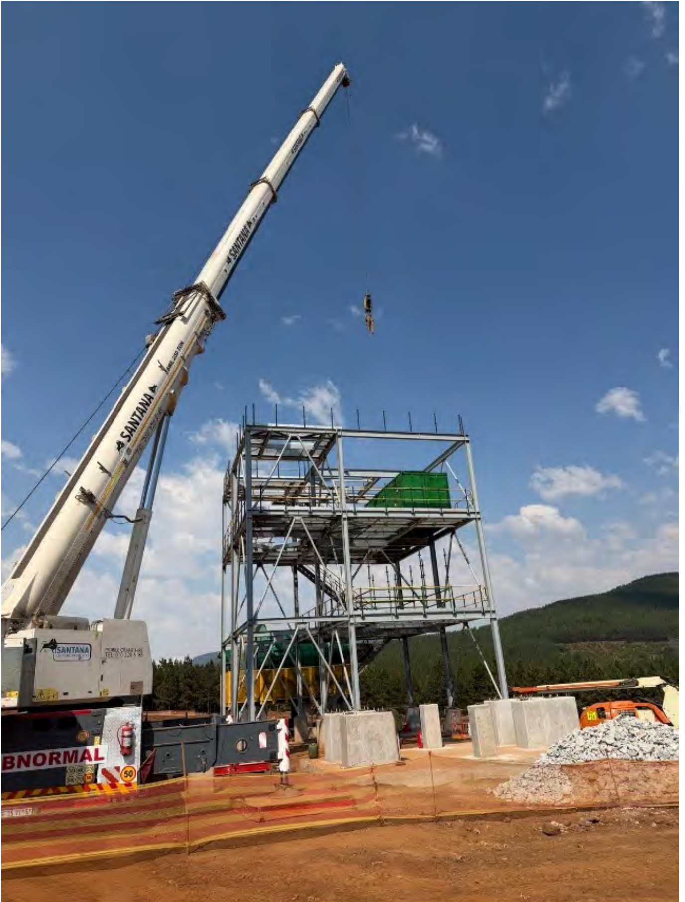
Figure 17: Ball mill plant construction in progress
