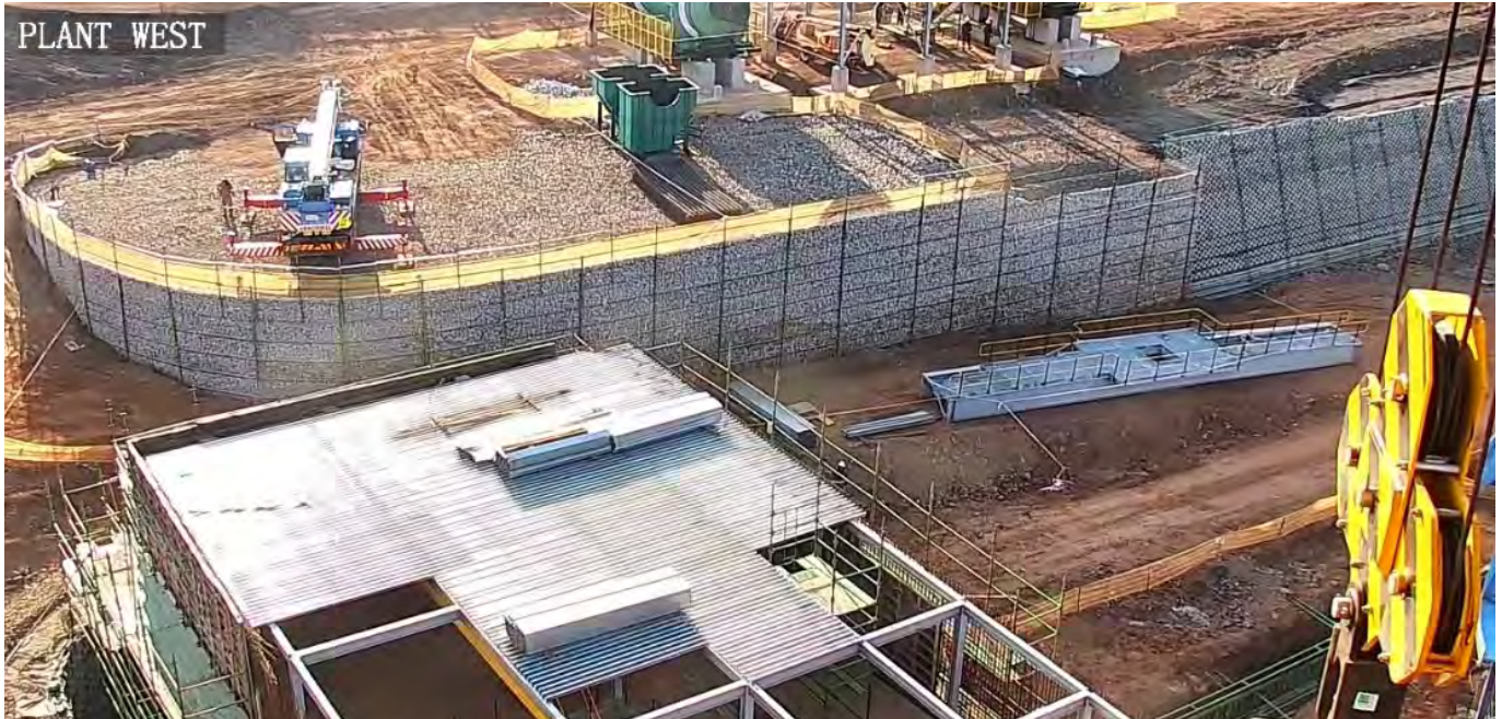
Figure 24: Gold Room Foundations
