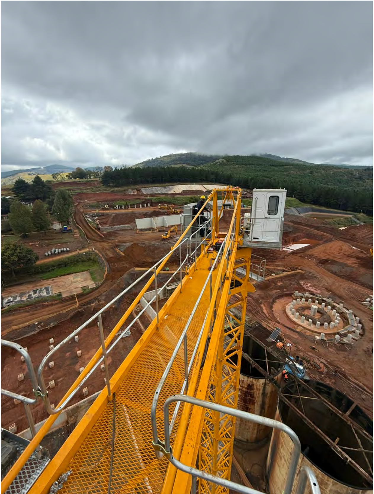
Figure 37: Tower crane installation and ongoing processing plant construction works
