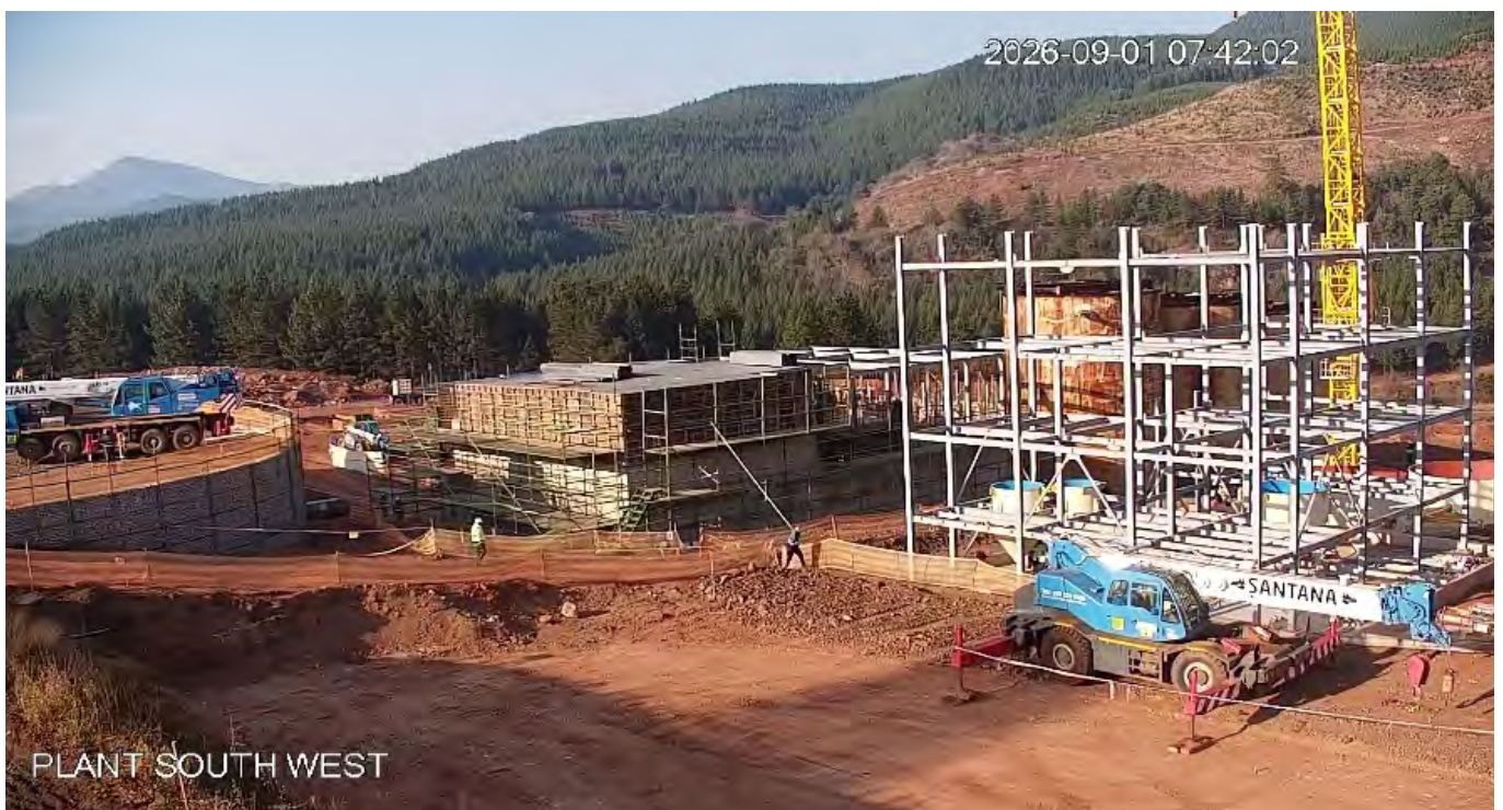
Figure 16: Elution circuit construction in progress
