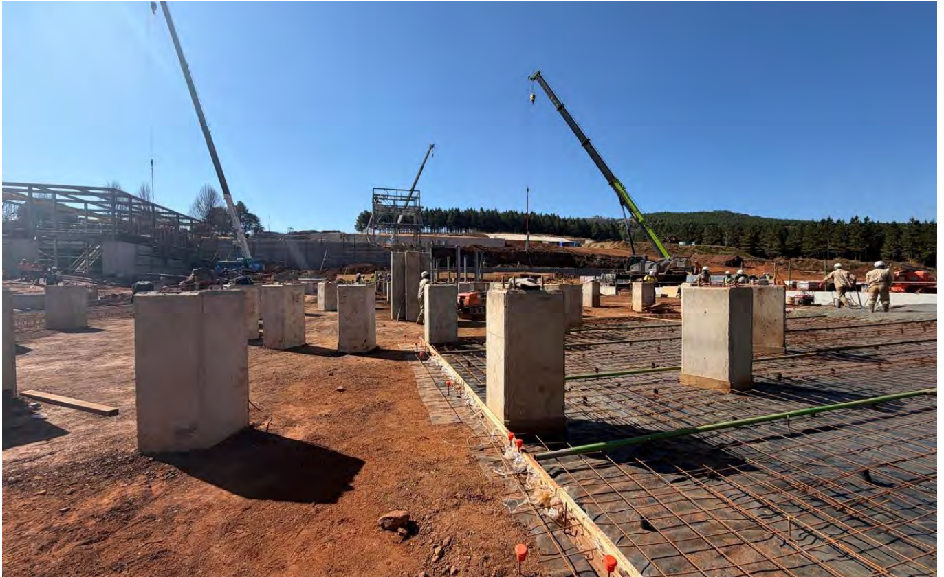
Figure 15: Concrete foundation works completed for the CIL plant
