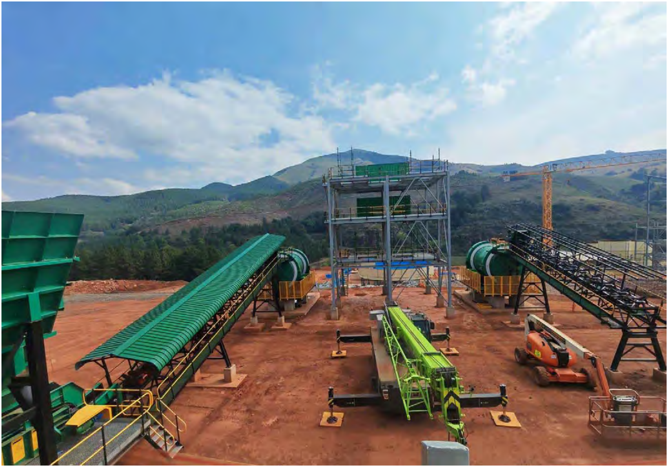
Figure 28: Installation of Twin Ball Mills
