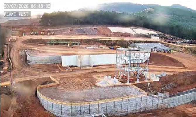
Figure 2: Construction of earth works and terraces at site
