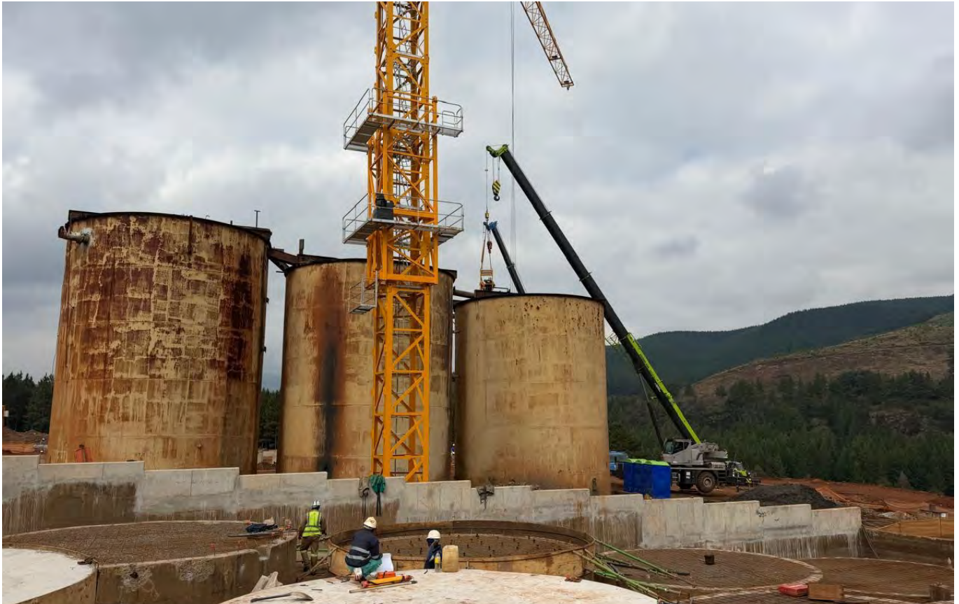
Figure 18: Refurbishment works underway on oxidation tanks
