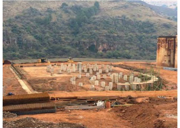
Figure 7: Thickener tank/processing area foundations
