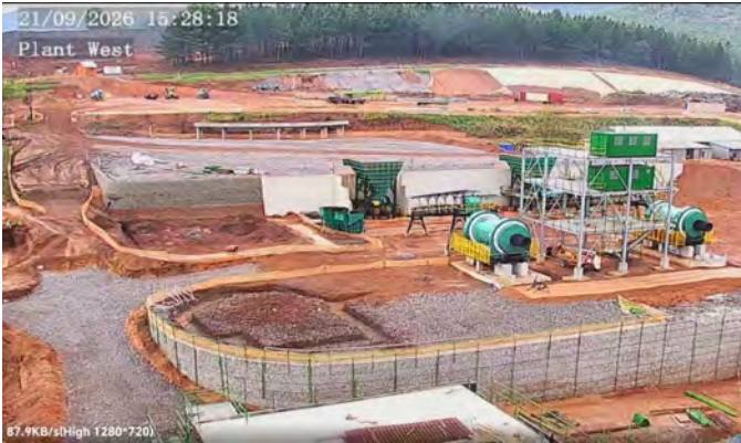
Figure 3: Ball mill and milling circuit construction advancing within the processing plant area
