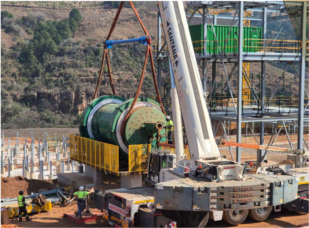
Figure 38: Placement of a ball mill during construction of the processing plant comminution circuit
