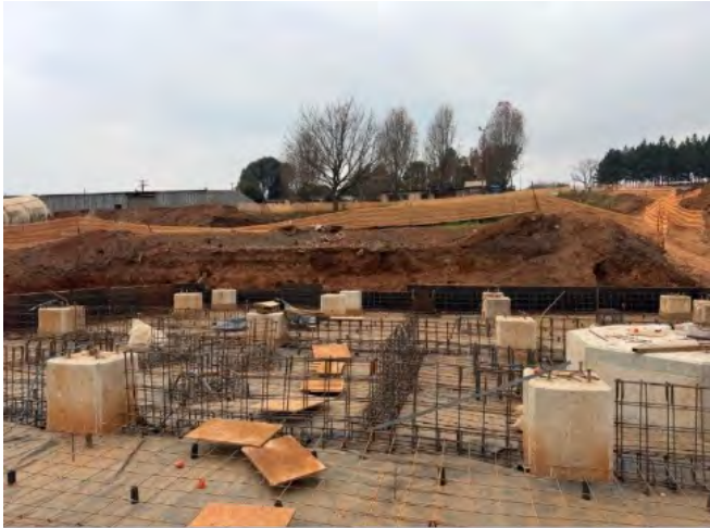
Figure 6: Elution circuit foundations
