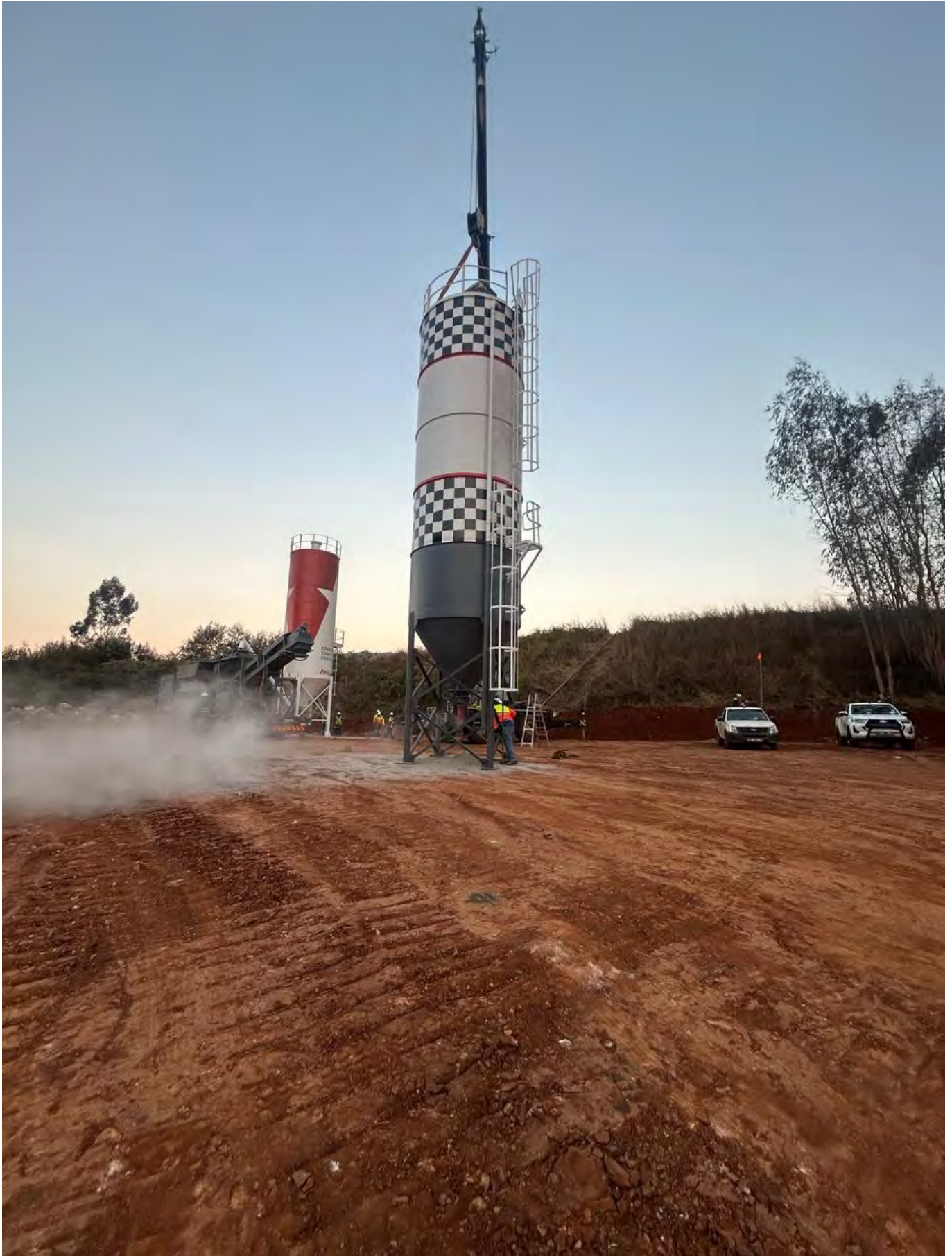
Figure 14: On-site concrete batching plant established to support project construction
