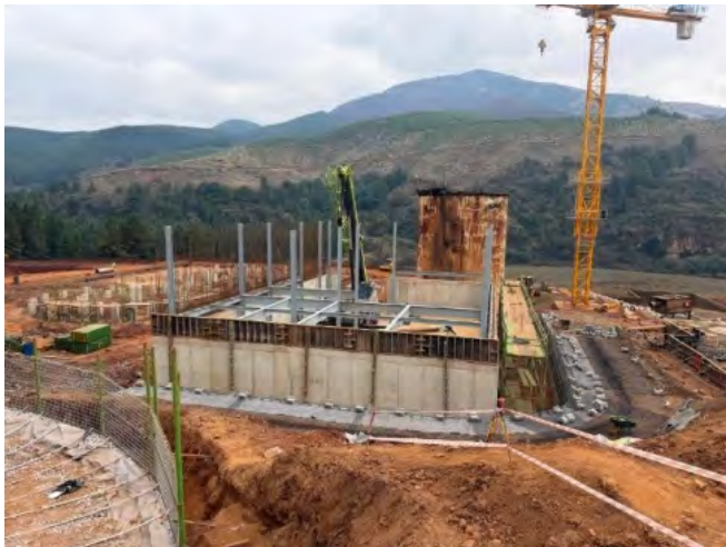
Figure 8: Gold Room construction continues - steel works
