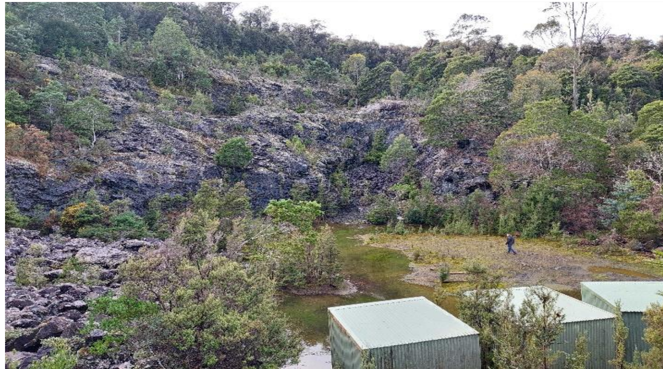
EXISTING HEC QUARRY AREA PROPOSED FOR THE PORTAL
