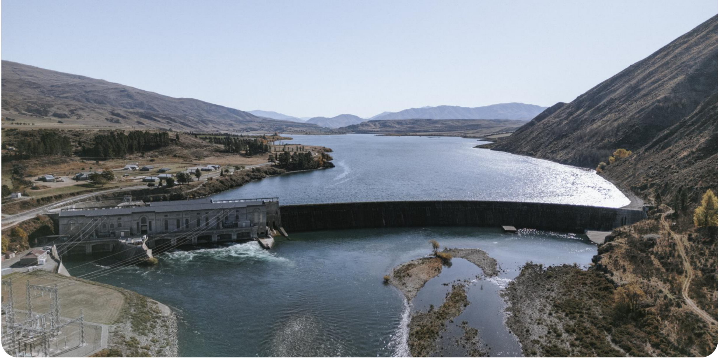
Construction of the Waitaki hydro power station originally began in the 1930's.
