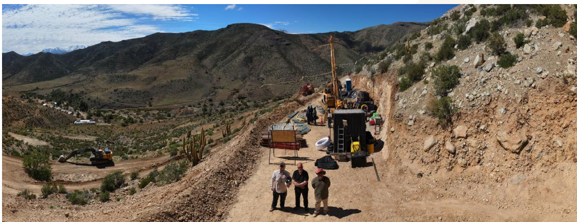
Figure 1. Diamond drill rig and support equipment at Ferro South, Llahuin Project, Chile
