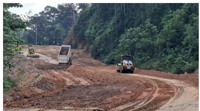
Road Widening, filling and compacting Segment B2
