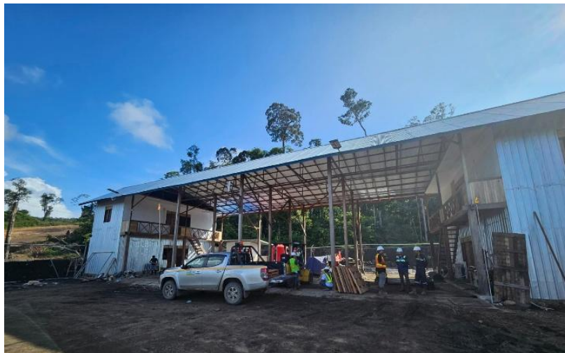
Drill & Blast Workshop
