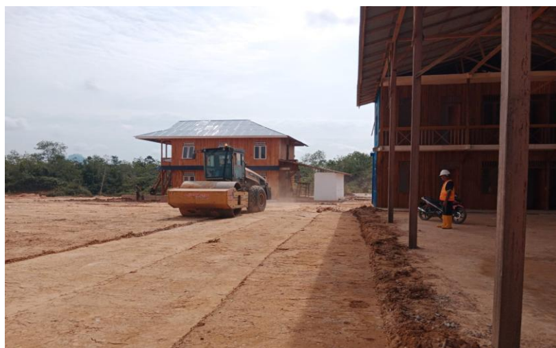
Additional Workers Camp and Workshop at Batu Tuhup Jetty
