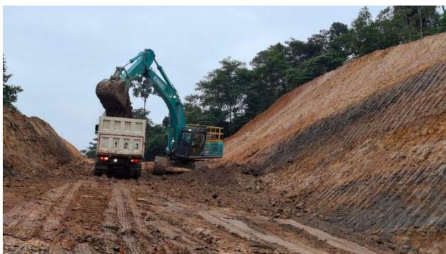
Wall sloping and road widening segment B2
