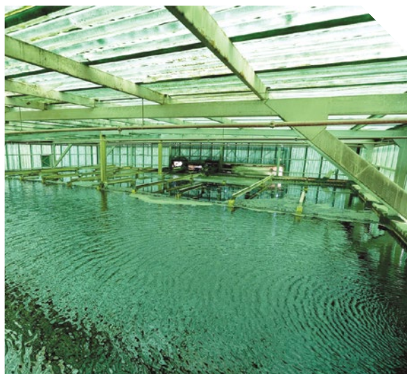
Solvent extraction circuit, Sierra Atacama processing plant
