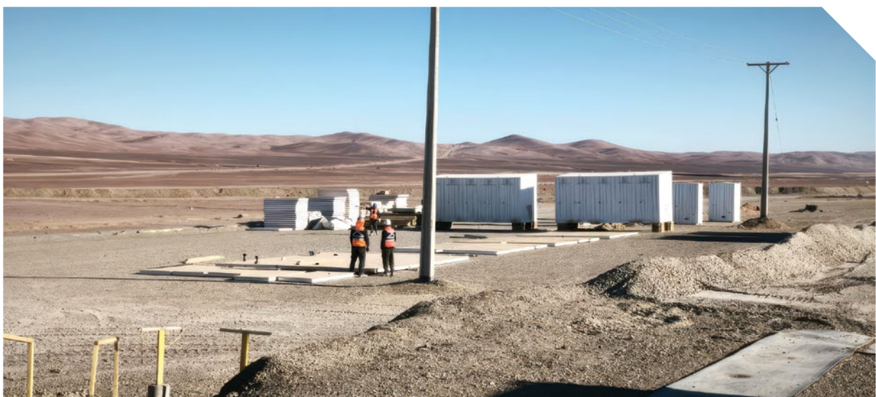
The exploration camp under construction
