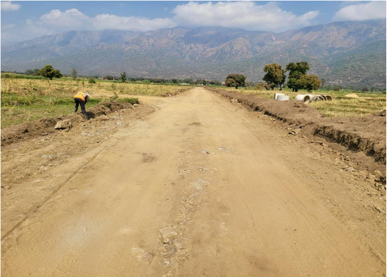
Figure 4. The newly constructed access road to Kinambo-2 is now complete and ready for operational traffic.
