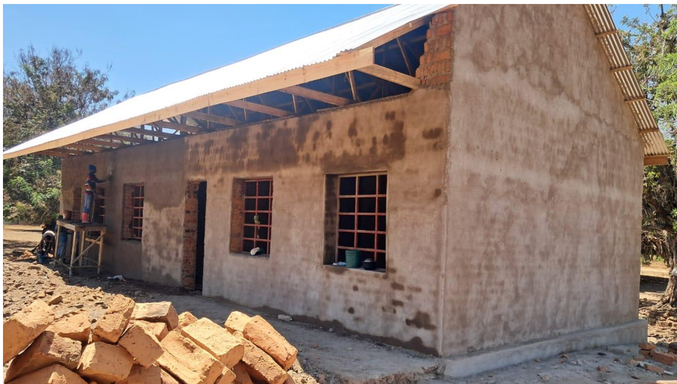
Figure 7. Kinambo village ongoing construction of the classroom
