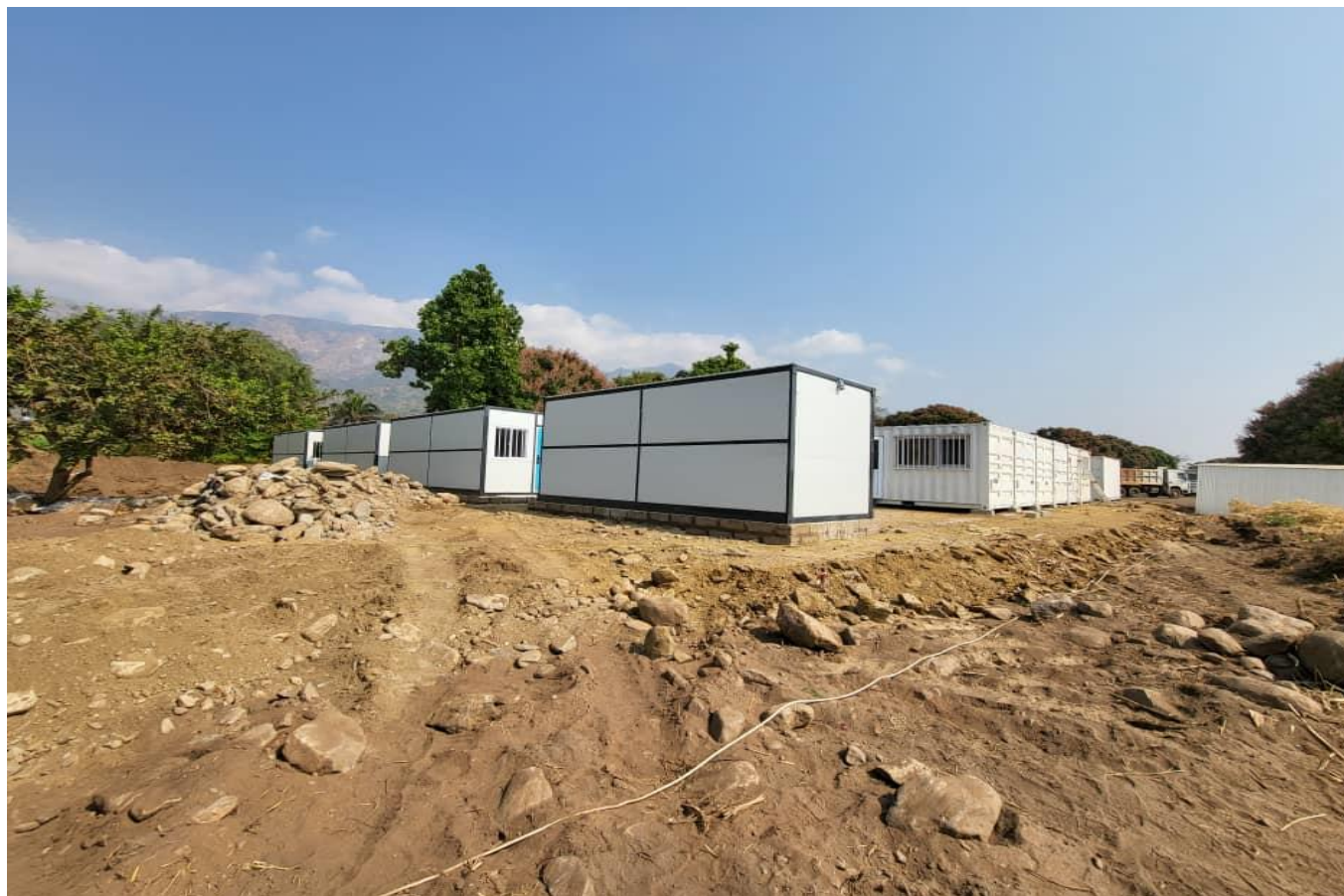
Figure 5. Construction and commissioning of a camp for 56 personnel is complete
