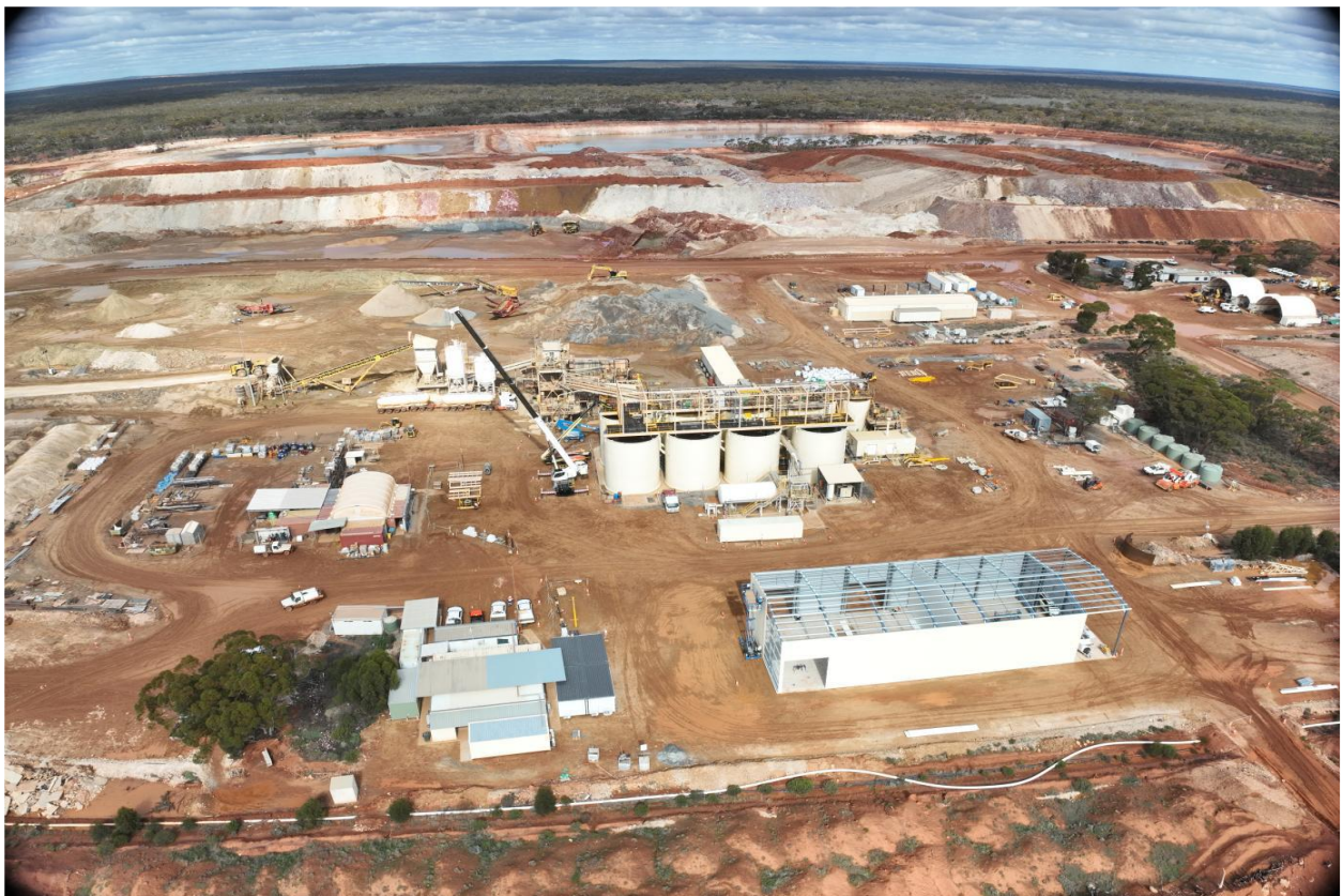
Image 5: Jaurdi Gold Project Mill Upgrade 28 July 2026
