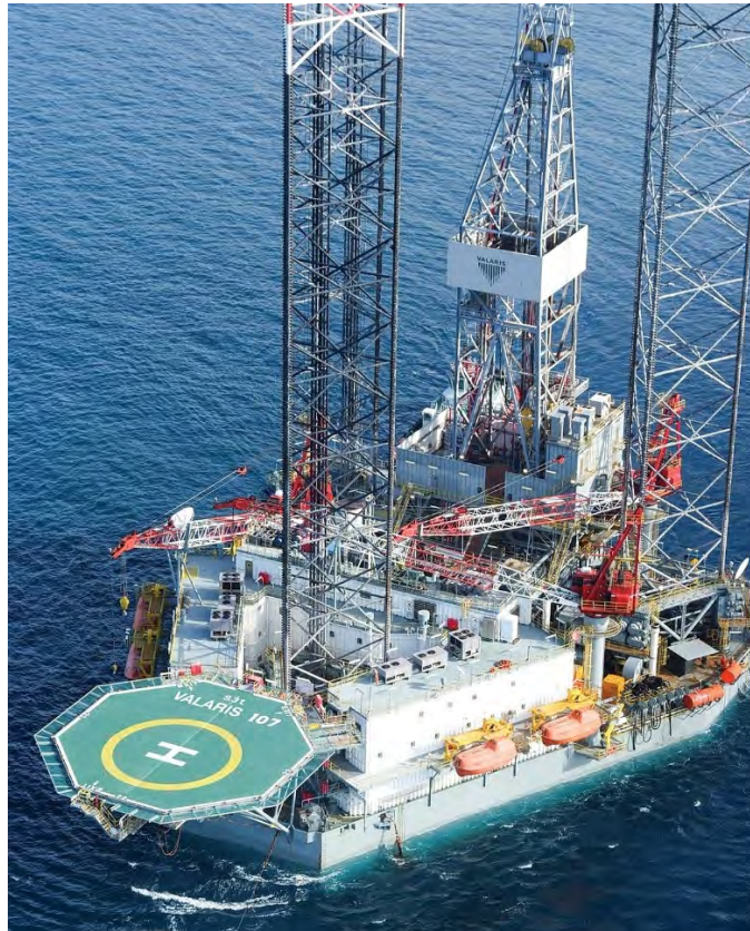
Figure 3: Valaris-107 Jackup Drilling Rig
